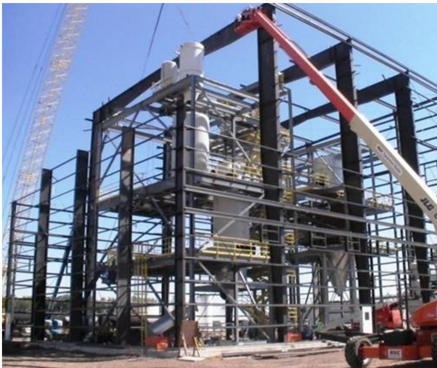
Photo 26 100 tpd Biomass Gasifier under construction (courtesy of Frontline)
