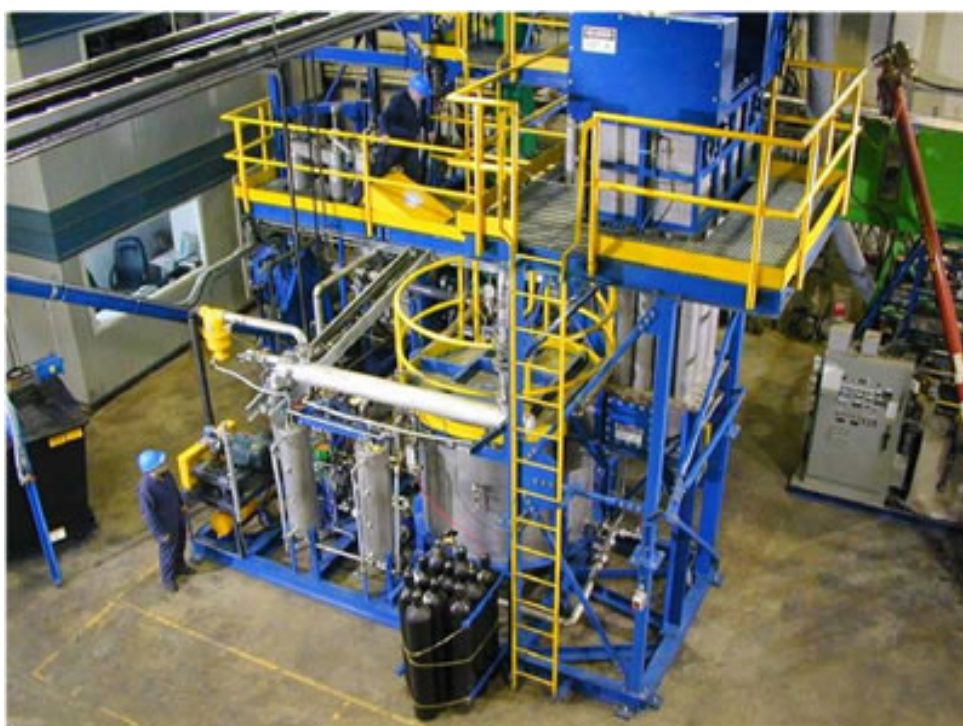
Photo 24 Dynamotive 10 tpd demonstration plant (from Dynamotive website)
