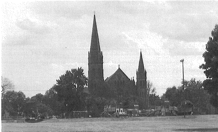
Photo 6: Holy Rosary Catholic Church, located on the southwest corner of 24 th Street East and 18 th Avenue South, across from the existing play area.
