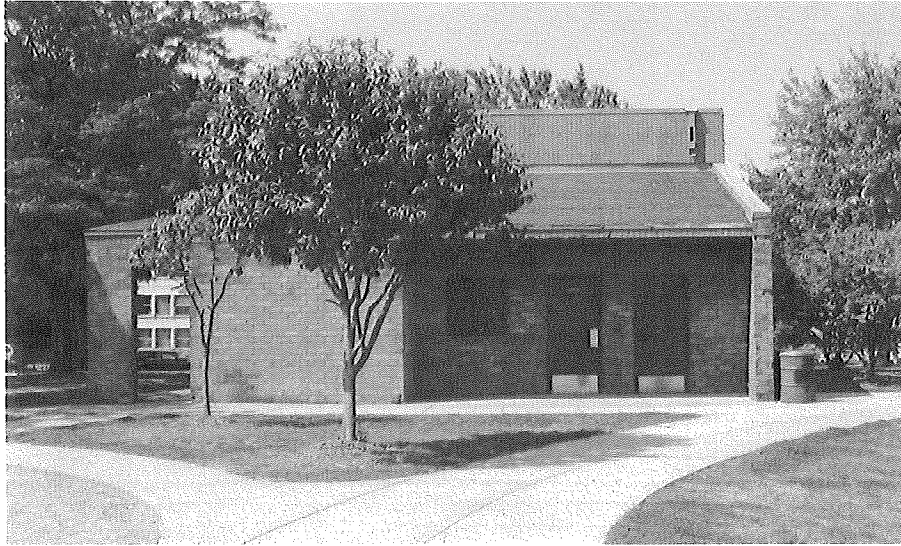
Photo 1: Park-side (east) facade of existing toilet/pump house building scheduled for demolition.
