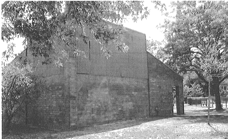
Photo 2: Street-side (west) facade of existing toilet/pump house building scheduled for demolition.
