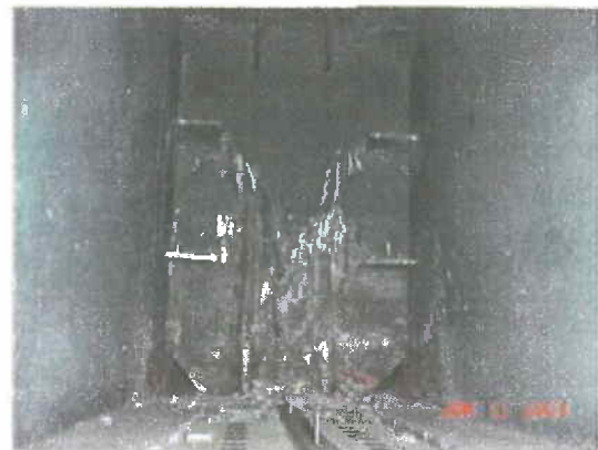
Front Side of Internal Diaphragm (Weld Tabs)
