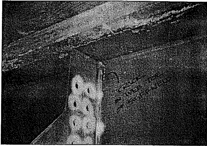
Girder #10 Vertical Stiffener/Girder Web
