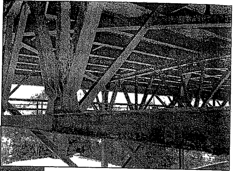
Bottom Floorbeam Truss Condition
