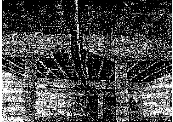
Multi-beam Spans Looking South
