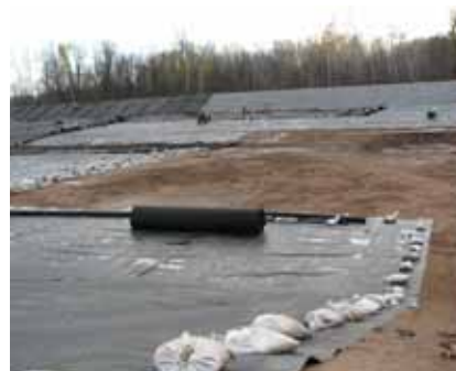
Laying Base Liner at Mille Lac's County Landfill
