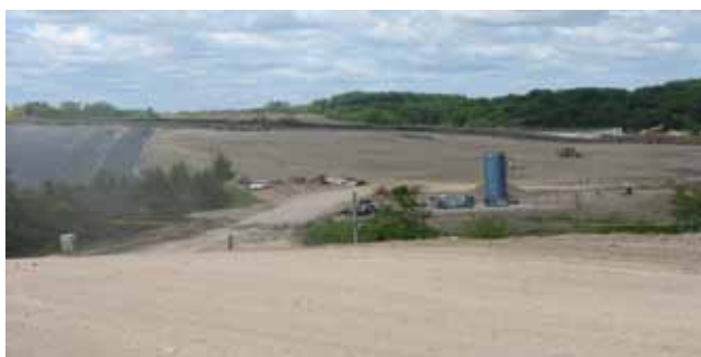
New Flare and Liner Construction at Woodlake Landfill, Hennepin County
