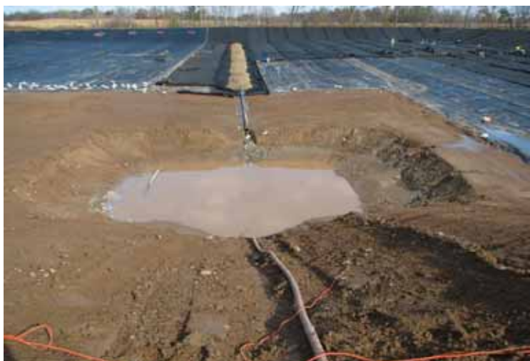
Constructing bottom liner and sump at Mille Lacs County Landfill
