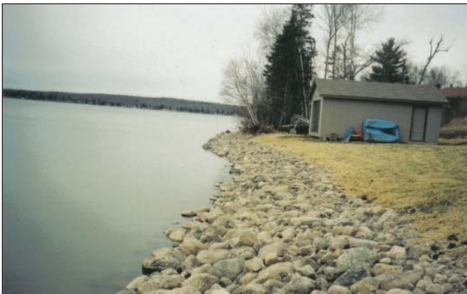
Pictured: Rock rip-rap shoreline protection project on Tulaby Lake.
