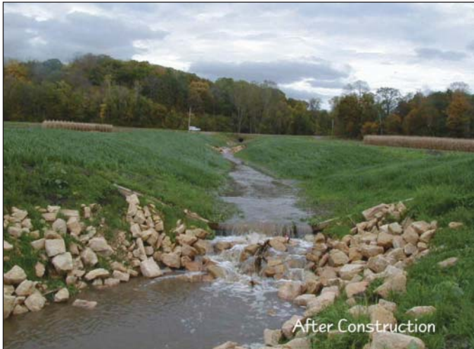
Pictured: This streambank stabilization project repaired a water body that was sending 255 tons of soil through erosion each year into the Minnesota River.
