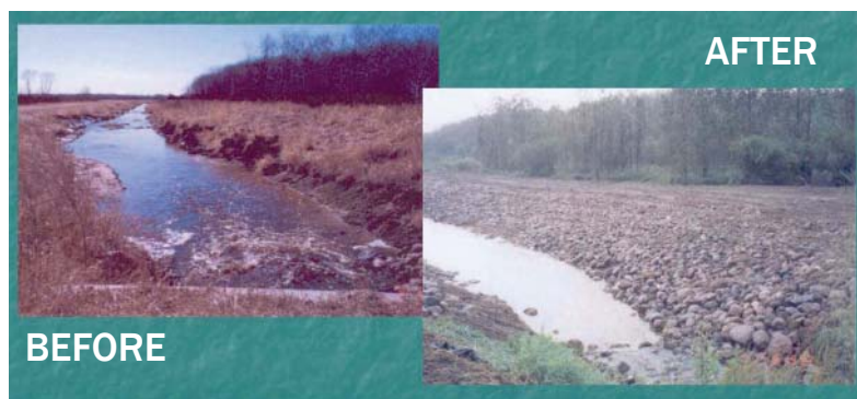
Pictured: The SWCD re-sloped and stabilized both banks of the Moose River near the impoundment outlet.
