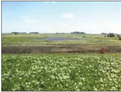
The black horizontal strip visible behind the orange tile inlet pipe is the ridge of a water and sediment control basin in this field. Parallel ridges are spaced 180 feet apart and help protect a CREP wetland restoration below.
