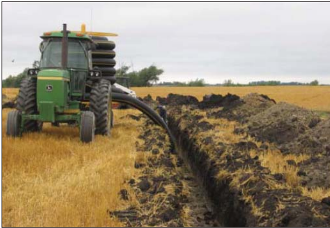
Pictured: Tile being installed as part of a sediment basin project.
