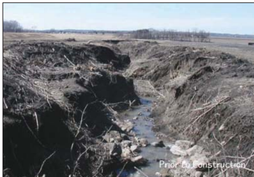
Pictured: This streambank stabilization project repaired a water body that was sending 255 tons of soil through erosion each year into the Minnesota River.
