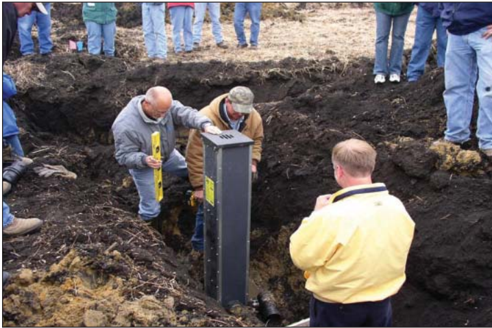
Pictured: (Above) Installation of a water retention structure for a controlled drainage project and (below) a wetland restoration project funded through CREP II.
