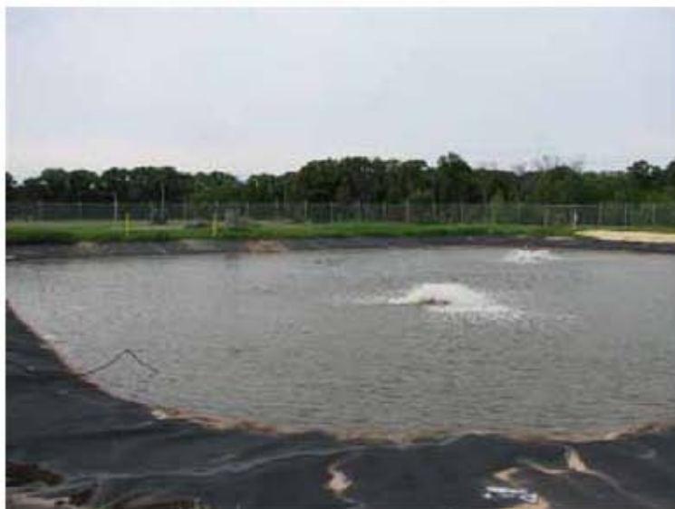
Ground water Treatment Pond East Bethel Landfill Anoka County
