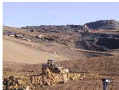
Waste relocation at the Winona County Landfill
