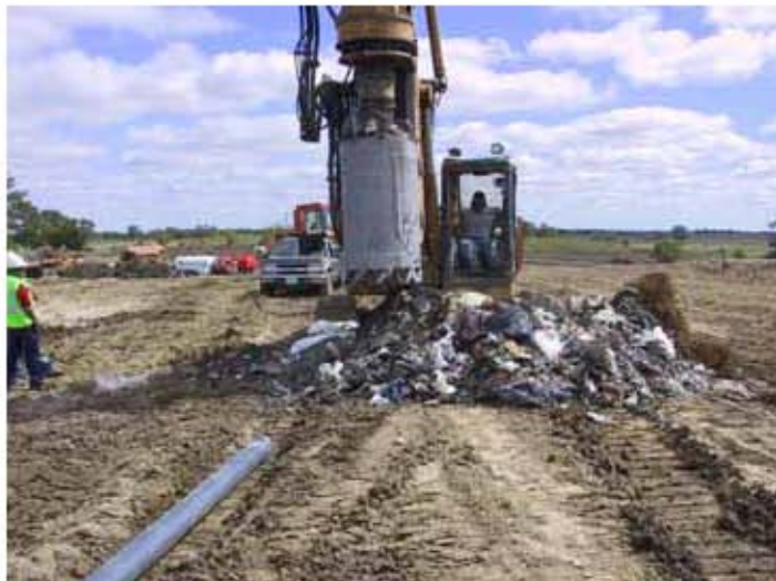
Drilling for Gas Vent Installation Meeker County Landfill, Meeker County
