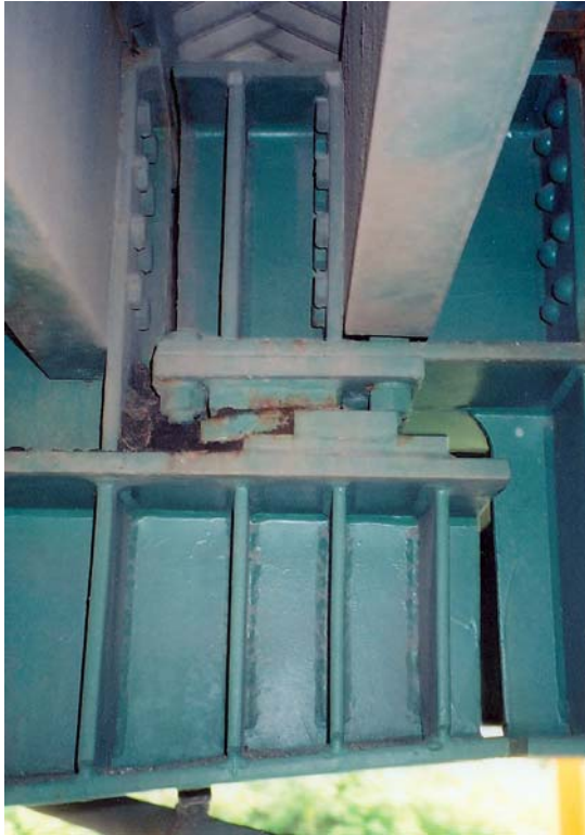
Sliding Plate @ Beam 5 NBL
