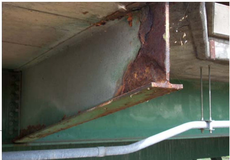
North Support Beam Stringer
