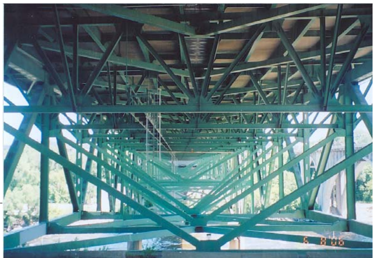
Deck Truss Looking North
