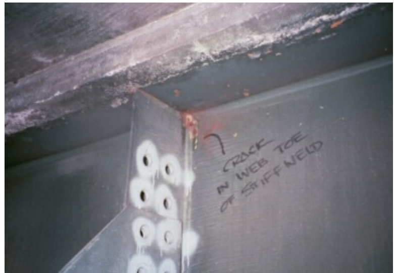
Girder #10 Vertical Stiffener/Girder Web
