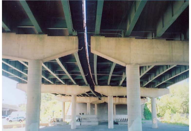
Multi-beam Spans Looking South
