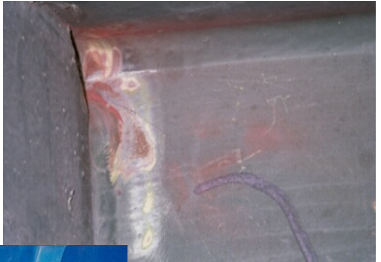
Girder #10 Vertical Stiffener/Girder Web
