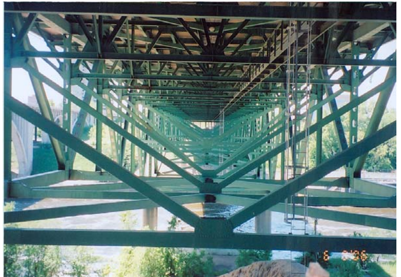
Deck Truss Looking South
