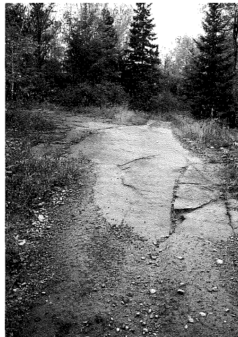
Rock outcrop crests are very desirable because they add interest to the trail, are very stable, and are essentially maintenance-free.
