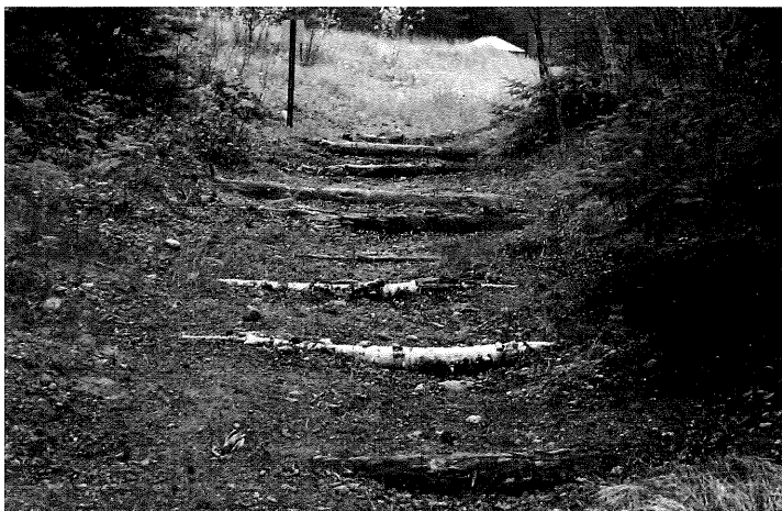
Trees are used as check dams to reduce erosion down this decommissioned, gullied, fall-line trail until vegetation is firmly established.
