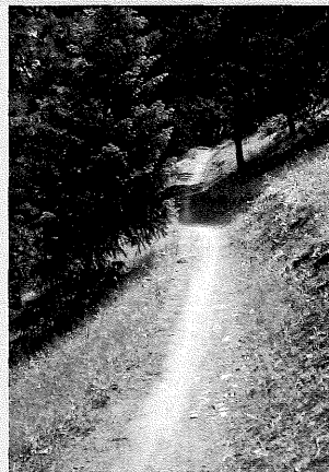
Jogging, climbing. The trail jogs up and down the sideslope as it gently climbs. Widely spaced crests and dips form fail-safe, highly effective crest volumes. (Mountain bike trail)
