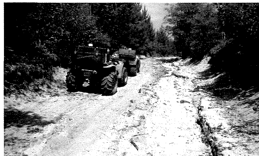
Fall line alignment, uncohesive soils. Continual road grading to remove erosion gullies from this steep forest road and snowmobile trail made the road 3 feet deep before it was traveled with ATVs. Note the ongoing erosion at center right.
