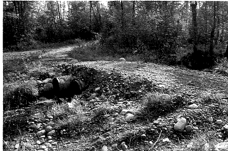
Acceptable. Culverts are embedded in a crest to cross a shallow channel. Note the thick tread fill with larger cobbles above the pair of culverts. Ideally, however, a substantial stream crossing would use a bridge rather than culverts.
