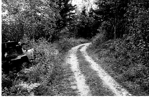
This trail is rolling grade on sideslope. Very desirable and easily sustained (downhill is to the left). Much of the roadway, cutslope and fillslope are overgrown, increasing both sustainability and trail experience.
