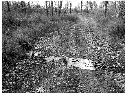
Low-speed, low-flow crossing. Class 5 plus larger cobbles cross this drainage on a forest road and on-road trail. With a seasonal flow that washes away small particles, the cobbles help reduce displacement and provide the tread surface.
