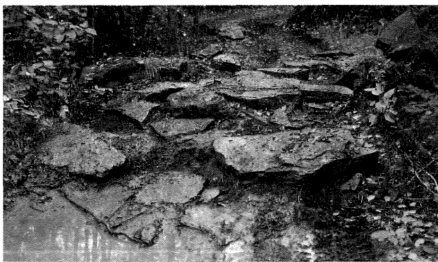
Reinforced constructed crest. This rock pile serves as a constructed tread crest on the Lower Money Talks off-road truck trail at the Iron Range OHV Recreation Area. The rocks serve double duty by challenging trail users while at the same time reinforcing the top of the crest against displacement. The crest prevented the water in the lower left corner from continuing downhill along the tread.
