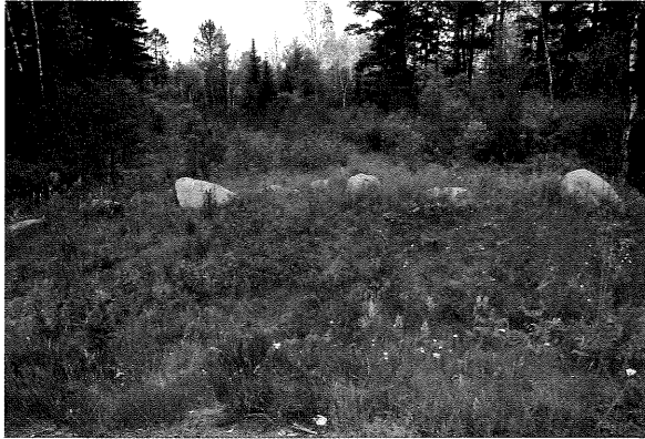
A road closure berm with embedded rocks has prevented traffic from entering this closed trail. Planting trees on the berm would help even more. Behind the berm, the forest is filling in through natural processes.
