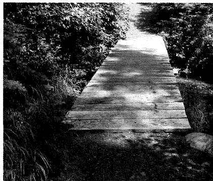
This simple, low-profile crossing is located along a more popular trail. A 60-inch width is justified so people can pass each other while crossing the drainage.
