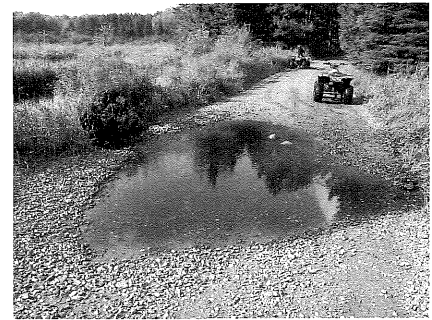
Ponding caused by displacement. Class 5 by itself does not withstand displacement with higher water flow rates – the particles are too lightweight. The higher the flow and the longer the period of flow, the more large cobbles are needed.
