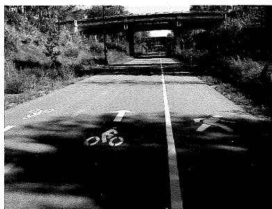
A solid white line may be used on a shared-use path to separate uses, with a broken yellow line used for separating opposing lanes. Pavement markings clarify proper uses and direction.
