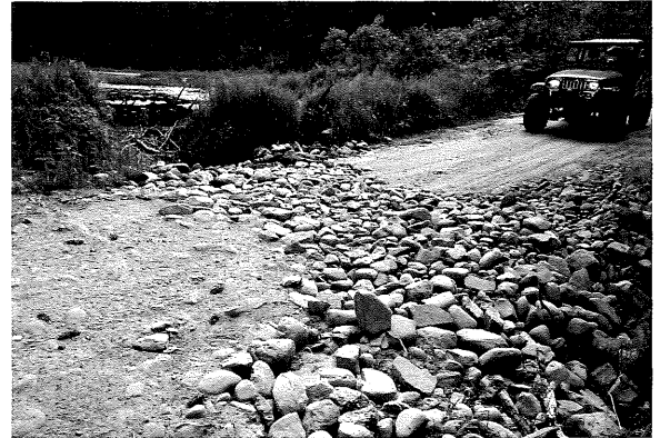
Cobbled overflow drainage crossing. This crossing handles wetland overflow when necessary. Because it is a floodway, geotextile beneath the cobbles adds resistance to scouring. Note the dip in this forest road.
