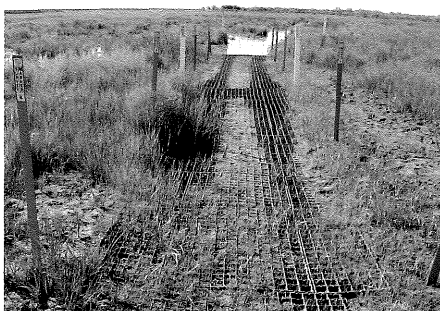
Green hardening. A major advantage of plastic porous pavement panels (top) is their ability to support vegetation. Each cell has a relatively large hole in the bottom through which vegetation can grow. This enables a drainage crossing to support plants even while serving as part of the trail.
