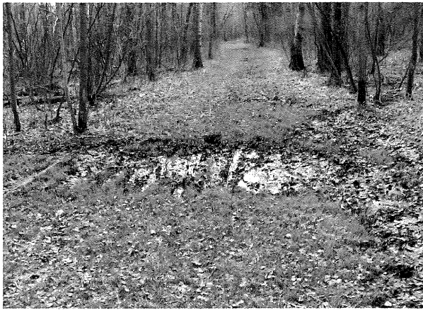
Problem: Perpetual seepage. This seepage/drainage area is a growing problem and will continually push trail users farther toward the edge, causing trail creep. A simple boardwalk could remedy this situation.
