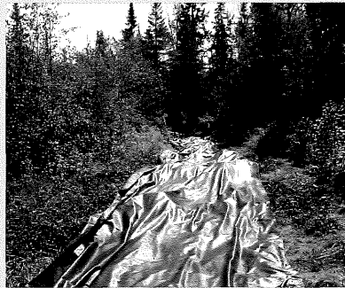
Geotextile laid before fill material is placed to create a stable trail tread through a stretch of unstable soil. Geotextile strengthens the tread and prevents the fill material from mixing with the soil below.
