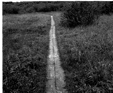
A simple boardwalk is often sufficient to provide trail access through a wetland with limited impact. In this case, there were no other options available to get through a 300-foot section of a trail that is 15 miles long.
