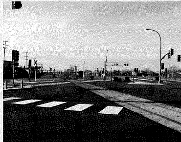
This rail crossing is at an odd angle and could result in a bicyclist catching a wheel while watching for motorists. The formed concrete with steel frame crossing helps limit the chance of that occurring.
