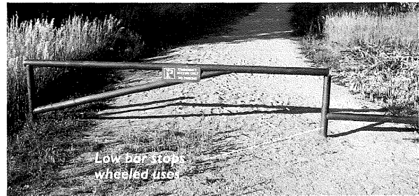
This modified stock gate excludes off-road trucks but allow ATVs on this on-road trail. The entire gate is opened for snowmobile use in winter and for timber management access as needed.
