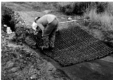
Green hardening. A major advantage of plastic porous pavement panels (top) is their ability to support vegetation. Each cell has a relatively large hole in the bottom through which vegetation can grow. This enables a drainage crossing to support plants even while serving as part of the trail.
