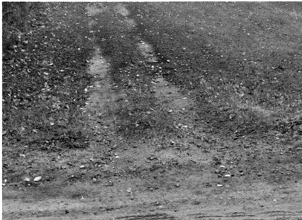
Problem: Growing impact to driveway approach. One of the most pressing concerns associated with forest access routes and right-of-way trails is the impact to driveway and road approaches. This example is close to the threshold for being unacceptable. If it gets worse, closure of the route by the local government engineer is likely.
