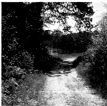
Narrow clearance. This sandy, low-use on-road trail remains sustainable because of low grades and narrow side clearance that tends to reduce speeds.
