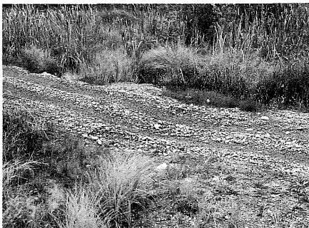
Typically dry equalizer drainage crossing. Class 5 plus larger cobbles stabilize this dip on a former railroad grade across wetlands.
