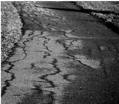
This trail, which is only 3 years old, illustrates poor pavement design and construction. Although initial costs were less than they would have been for a heavier design, increased maintenance and short design life make long-term costs much higher. Of equal importance, the user experience is diminished because the trail becomes rough and hard to walk, bicycle, or in-line skate on.
