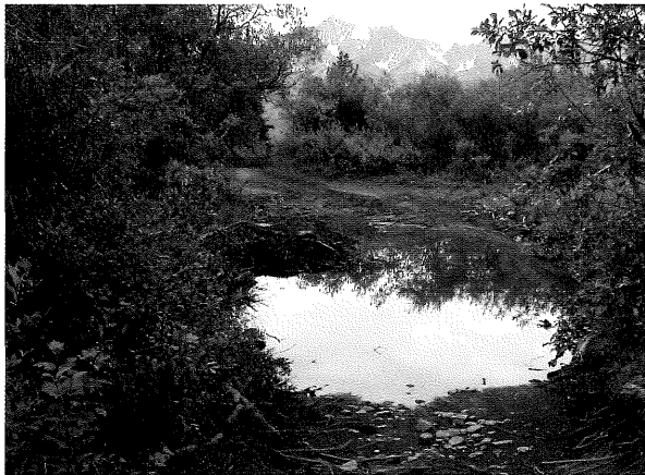
Problem: This ATV trail goes across a shallow drainage that has been deepened through use. This will continue until the hole is too deep to go through, which will force riders to bypass the area, which will cause further problems. Proactive rerouting is the best solution, although closure might be necessary if the problem is persistent in the area.
