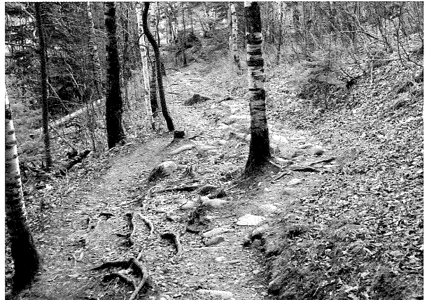
Problem: Bypassing trail protrusions. Even a few rocks and roots in a hiking trail can entice trail users to find another route. Left unchecked, this type of activity can slowly detract from the trail experience and the natural setting. Stronger anchors (and "stay on trail" signs) are needed to keep this from getting worse.
