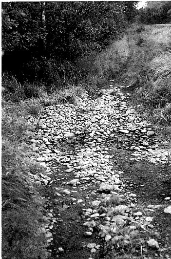
Cobbled crossing of a wetland drain. On this ditch trail, cobbles were used below the road culvert to provide a stable, nonmuddy crossing for ATVs. The usual ATV displacement is not a problem because water flows between and over the stones.
