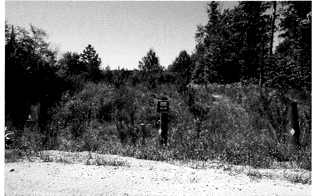
This recently constructed berm closes a rerouted trail. Conifer seedlings were planted behind and on the berm. The sign reads, “Seedlings Planted – Keep Off” and the tops of the wood posts are emphasized with red paint. This berm has kept motorized traffic out of the closed area.
