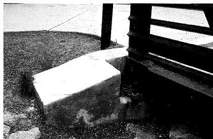
When a bridge can begin at the top of a slope, the visible portion of the headwall will be very small and pose minimal impediment to flooding. Note how the abutment is widened and the top sloped to serve as a retaining wall for the trailbed.
