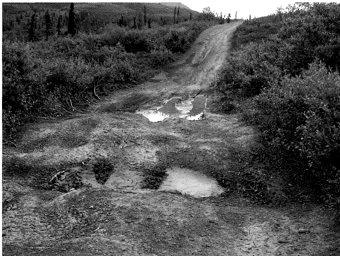
Problem: Trail sprawl. If seemingly minor holes and ruts are left unchecked, it is inevitable that a trail will keep expanding and/or new bypasses will be created. These problems are common in areas of organic soils and solving them is no small challenge. Avoiding organic soils is the best solution. Where that is not possible, careful alignment using rolling grade techniques and site anchors to keep riders on the trail can help curtail problems.
