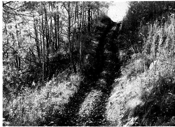
Problem: New trail too steeply traverses a rocky slope. The trail will capture all of the rainfall on the tread, plus that from the slope above it (right). This will cause unsustainable erosion and, ultimately, the trail will have to be redesigned.
