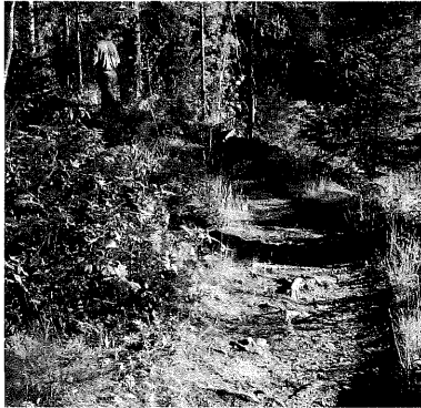
Foot tread. Compaction and displacement from extensive use deepened this tread. The compacted tread is firm. Some soil loss is due to erosion from water flowing down the trench initially formed by compaction and displacement.
