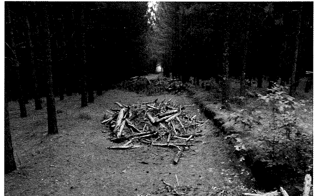
In addition to a closure berm, this road/trail was also closed with intermediate berms and slash. This is most effective in heavily wooded areas where off-trail travel is difficult.
