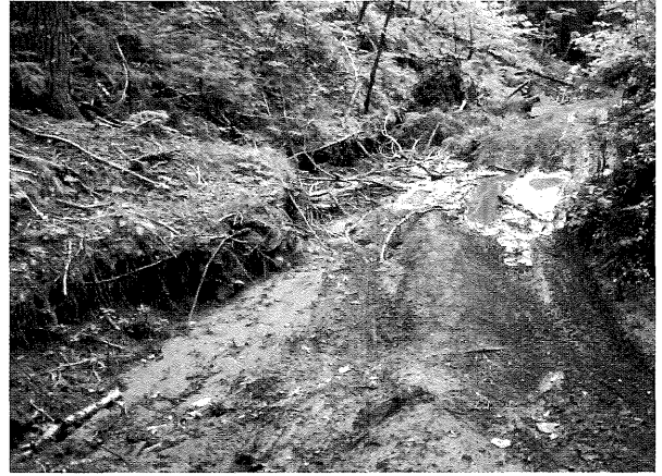
Problem: Severe soil erosion adjacent to a hillside due to poor trail design. This will indefinitely continue and cause increasing levels of downstream sediment. Rerouting or closure of the trail is mandatory.
