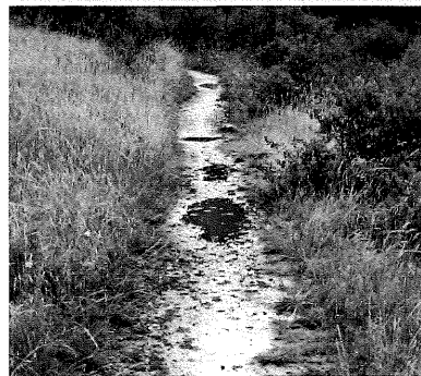
Compacted treads, with reduced air spaces between particles, are firmer and more resistant to displacement and erosion. But they also absorb less water, increasing the amount standing on or flowing down the trail. In this level area, water puddles on the tread, while it sinks into the ground everywhere else.
