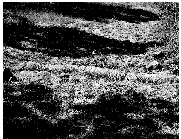
This straw wattle serves as a temporary device for slowing and diverting water.
