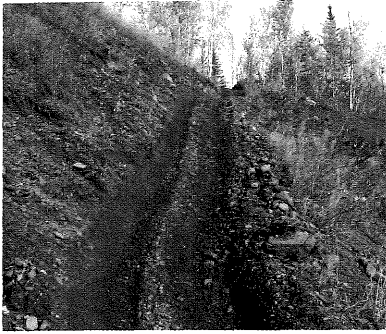
Edge protection. This ATV trail was intentionally formed with a bermed outside edge for safety. Vegetation will eventually blend the berm into the site, strengthening it in the process.
