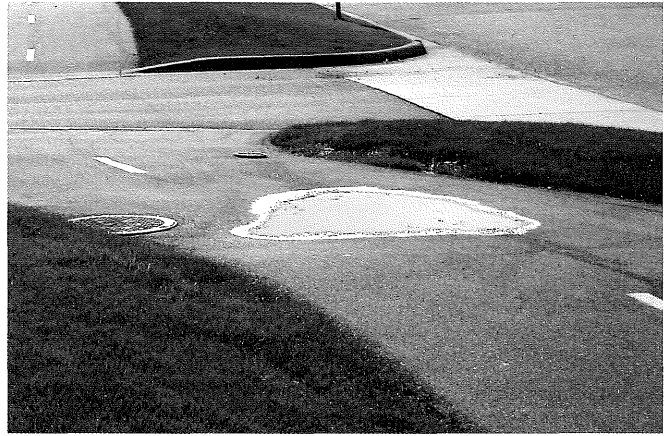
"Bird baths" are largely avoidable if the contractor is paying attention to subgrade preparation and cross slope prior to laying down the pavement. This dip should be corrected.
