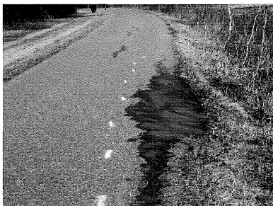
Without addressing the underlying problem, this edge patch will likely only be a temporary solution. It is also fairly rough, meaning that trail users will drift into the opposing lane to get around it.
