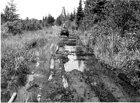
Problem: Compacted and displaced tread in lowland area makes the tread unstable. Attempting to drain this tread would drain the entire area, unacceptably changing the hydrology of an adjacent wetland. Rerouting or closure of the trail is mandatory.
