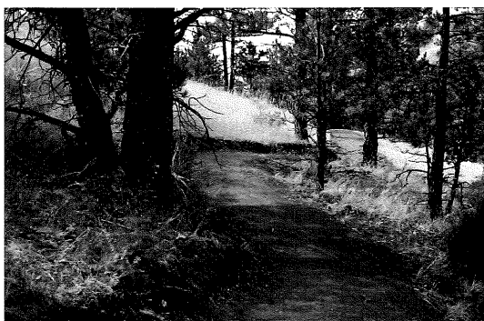
(Left) This trail climbs faster than it might appear. Rolling grade is used to limit tread watersheds on this erosive soil. With tree anchors, it is also used to make the trail more interesting to visitors.
