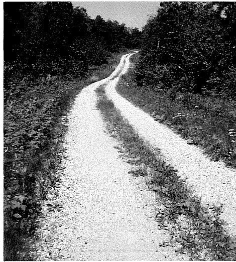
Soil variability factors into sustainability. Compactible soils, such as well-graded gravel (left), are best suited for natural trails due to their inherent stability. On these soils, displacement and rutting should be minimal. On sandy soils (right), more displacement can be expected and cause somewhat deeper ruts than would be expected in other types of soils. As long as erosion, migration of soil into water bodies, excessive rutting, and bypassing are kept in check, this trail can remain sustainable even though the tread itself shifts a bit over time. Trails on sandy soils generally require more monitoring and prompt action if a problem occurs.
