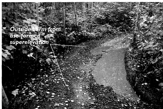
As both of these photos illustrate, superelevations can be formed through regular trail use by wheeled vehicles such as OHVs and mountain bikes.
