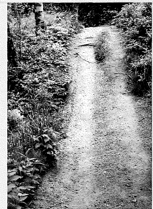
In-line, climbing. The trail rolls over a small natural ridge. This short, steep climb is sustainable. Small crests such as this are fun for wheeled uses. (Hiking trail, with ATV tracks from recent trail maintenance)
