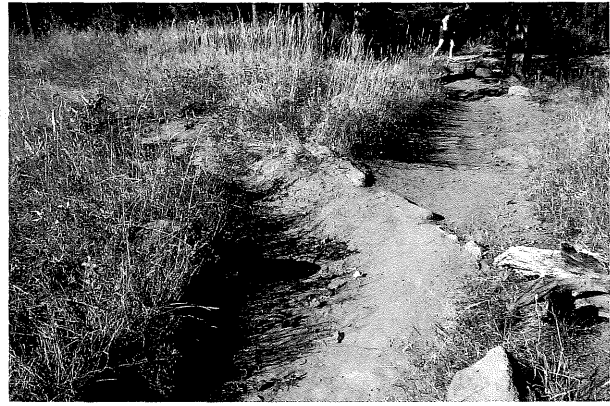
A stone waterbar with soil on the uphill side can be used on treads with low grades where the stones are too small or do not fit together well enough to form a free-standing face. Note the wide outlet and the smooth way water flows into and through it.
