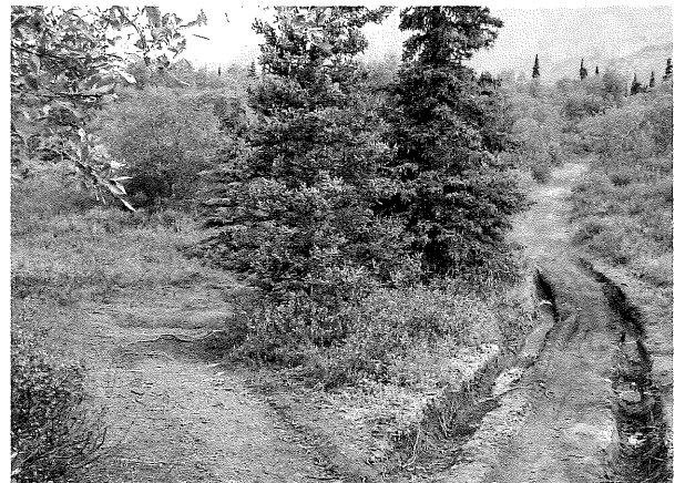
Problem: Bypassing. The deep rutting on the right encouraged riders to create a new route, which over time will also likely rut in these organic soils. Since this is a designated OHV trail, realigning the trail to higher and more stable ground is the best solution.
