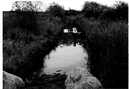
On level or near-level ground, compaction and displacement sink the tread below the surrounding soil level. The tread then ponds water, causing mud and mudpits.
