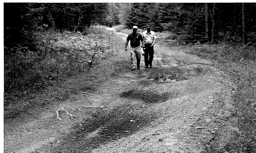
Excess clearance, excess sightlines. Too much clearance enables higher speeds with longer sightlines. This resulted in rapid tread displacement, as seen in the foreground. Having shrubs and trees next to the tread would improve the situation.
