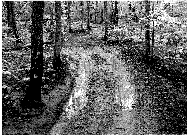
Problem: Compaction and displacement on a near-level site deepening the tread of this relatively new ATV trail. Water ponds on the tread because it is the lowest point. Fixing the problem by improving drainage and perhaps hardening the tread through this section are possible solutions.
