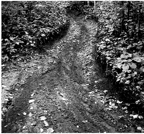
Problem: Excessive displacement. Heavy use, erodible soils, and lack of rolling grade have combined to excessively displace soils along this trail. Rerouting and/or closure is necessary since fixing this is almost impossible.
