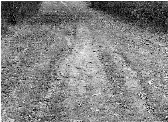
Problem: Lack of underlying soil stability. Organic soils are inherently prone to rutting. Although still within rutting limits, this trail is close to becoming unsustainable, especially if soils begin to migrate to adjacent systems and water bodies. If foot traffic is low, periodic reseeding and filling may be the best approach. If the problem continues, rerouting may be necessary.
