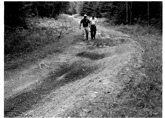
Excessive clearing along this forest road creates long sightlines, causing OHVs to travel at higher speeds and create displacement bumps.
