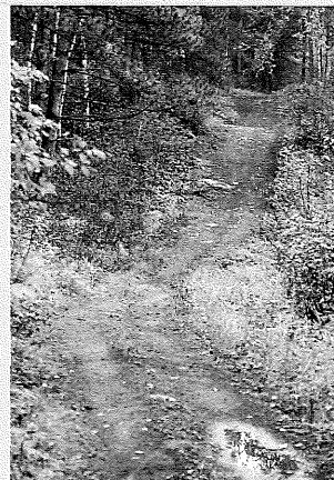
In-line, near-level. The trail flows over a series of natural crests in glacial terrain. With almost no sideslope, tread climbs follow local fall lines, limiting future drainage options. (ATV and snowmobile trail)
