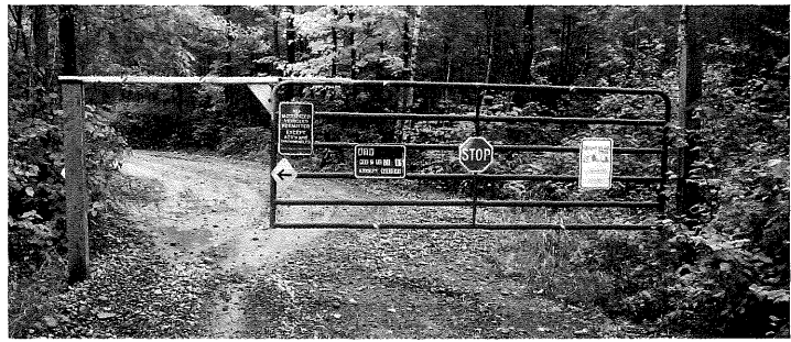
This modified stock gate excludes off-road trucks but allow ATVs on this on-road trail. The entire gate is opened for snowmobile use in winter and for timber management access as needed.
