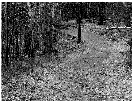
The nice even trail tread with a slight cross-slope is well suited for a two-track set through the woods, making for easy grooming and fun skiing.
