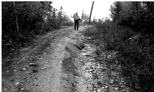
Fall line alignment, uncohesive soils. Even without trail use, this forest road used as an on-road trail would have severely eroded from being too steep in loose, sandy soils.
