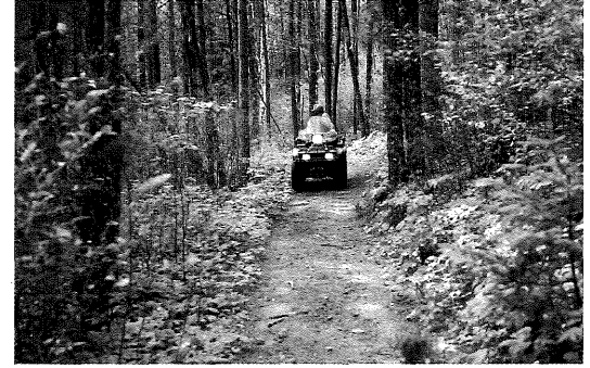
Hardened logging road with rolling grade. Overgrown now, this former logging road was partially compacted by logging equipment. ATVs consequently have little effect on the hardened tread.
