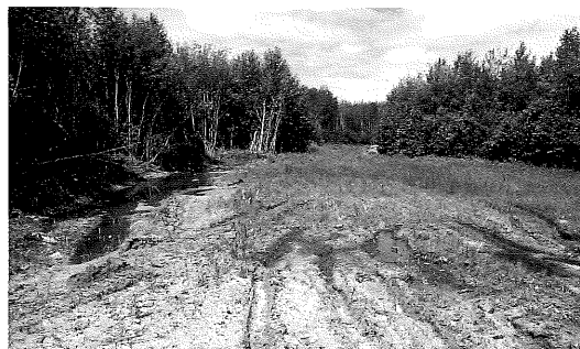
Level or near-level, poorly drained or uncompacted roads, skid trails and logging areas. Temporary forest roads in these conditions are usually unsustainable for trails unless elevated, hardened, ditched, drained, and maintained like roads.
