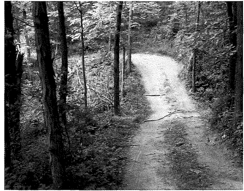
Given the compaction and displacement forces of OHVs, well-anchored and well-placed dips are necessary to prevent bypassing and excessive superelevations from occurring. Even these small trees help keep the user on the trail at this dip.
