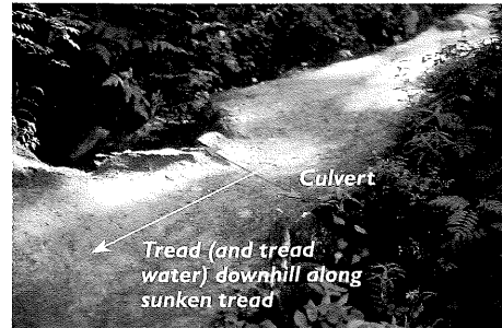
AVOID where possible. Although very nicely formed with stone headwalls and tailwalls, if this deep-channeled culvert were to clog, water would be diverted down the tread because there is no tread dip. Also note how tread wear has depressed the center of the tread, allowing tread water to follow the tread over the culvert.
