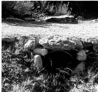
Optimal. The tread dips through a relatively deep channel, so the overflow flows over the tread above the culvert. Note the tread climbing on both sides.
