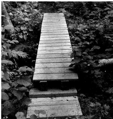
This simple drainage crossing was made from treated dimension lumber. The 24-inch width is appropriate for its level of use, where the likelihood of meeting someone at this spot is minimal. No handrail is needed since it is less than 30 inches above the ground.
