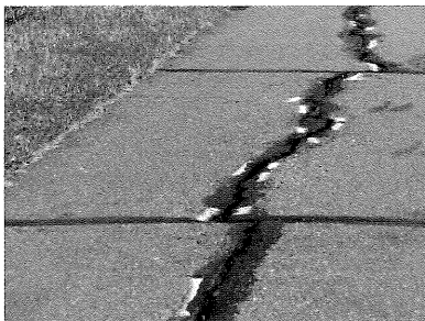
This crack is getting very close to being too wide for filling, with the next step being to remove and patch the area or do an overlay.
