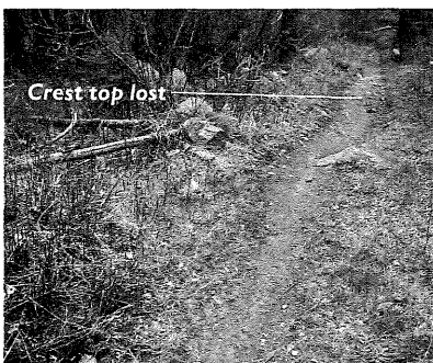
Displacement and compaction. This small former crest has lost its top to displacement and compaction. It was simply too small. A larger, longer crest would have lasted much longer.
