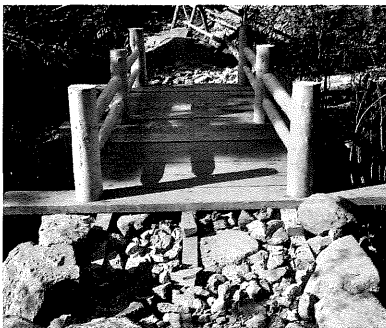
Seen under construction, the ends of three steel stringers (topped by wood nailing strips) are embedded in this unmortared stone abutment. Stone minimizes the footprint of the raised abutment while visually anchoring it. Rock fill provides excellent drainage and reduces settling and tread displacement.
