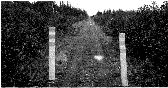
Removable bollards, padlocked at their base to pipe sleeves embedded in the tread, prevent use of this ATV and snowmobile trail by on-road vehicles. The reflectorized bollards are removed during snowmobile season.
