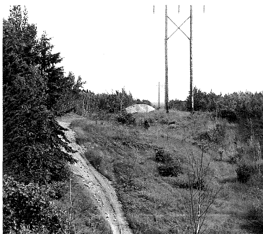
Avoid certain utility corridor roads, especially those that have unsustainable soils or alignments for trails, high runoff and splash erosion due to tree removal, and/or low stewardship value. This corridor road exhibits all three conditions.
