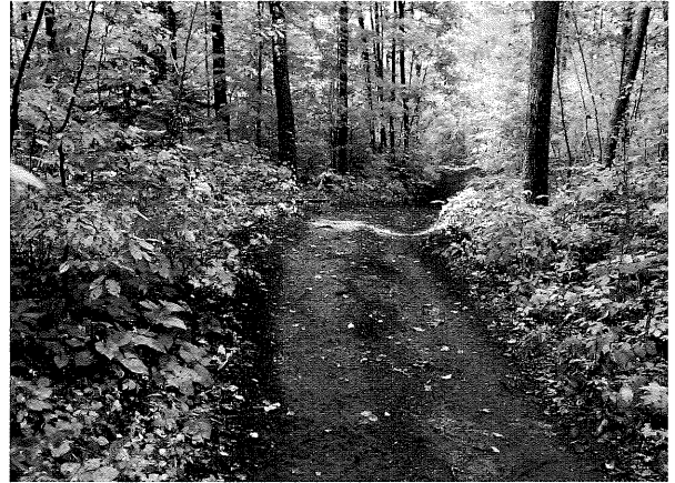
Rolling grade design and alignment ensures that this ATV trail will remain sustainable. If runoff is managed through dips and crests, erosion can be largely prevented with normal use.
