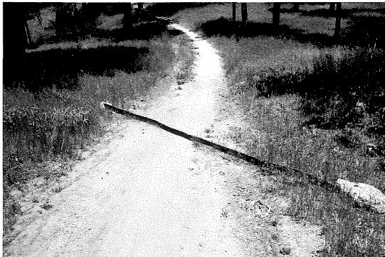
This highly angled flexible waterbar has worked well for years on this heavily used mountain bike, hiking, and horse trail. The trail is fairly steep, with a sideslope down to the left. Tread is firm and stable with low displacement. A very long bar, extended on both ends, with anchor rocks at each end effectively convince visitors not to bypass it. Mountain bikes have no trouble with the bar angle.
