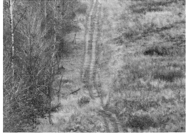
This rolling grade trail is both fun and sustainable, in spite of its heavy use. Notice how the dips and crests help manage stormwater and prevent erosion.
