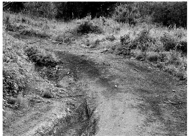
Problem: Severe, ongoing erosion on a modest slope. Disregarding the drainage characteristics of a site is a prescription for this kind of problem. This trail will have to be redesigned using rolling grade techniques if it is to be sustainable. Otherwise, closure will ultimately be necessary as the problem gets worse.
