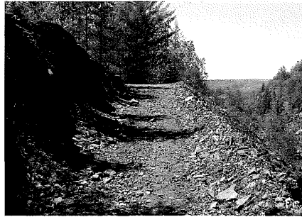
The trail is anchored by slopes and rock berms in this quarry site. The manipulation of the anchor is acceptable due to past site uses.
