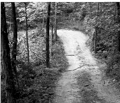
Correct drainage crossing. This ORV trail properly crosses a drainage swale by dipping through it and climbing on both sides. After climbing out of the crossing (background), the trail continues dropping while traversing the slope.
