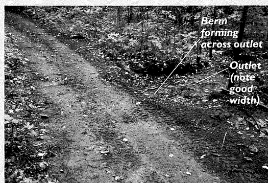
Dip outlet berming may still occur with high displacement uses, even if tread is straight. Outlet berms will still need to be removed during regular maintenance, and the dip and outlet should be formed to drain the tread even when a berm forms.
