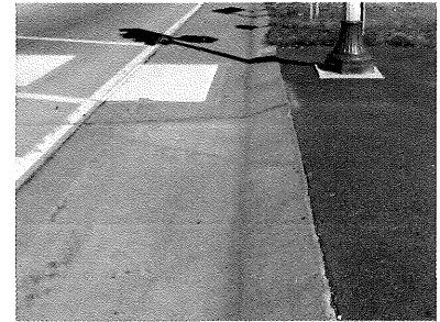
Users of this long crossing are met with a curb, not a ramp. This is far too abrupt and annoying to trail users trying to get across an intersection. The light standard in the middle of the path is also an unnecessary obstacle. It is not an accessible solution.
