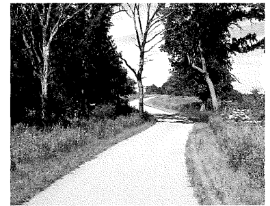
A simple curve introduced into a long stretch of trail will often cause travel speeds to go down. It also makes the trail more visually interesting.
