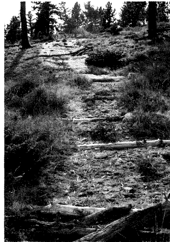
(Left) Scarification of a former compacted trail surface was mechanically ripped and topsoil and organic material from the replacement trail were added to partially fill the old tread.
