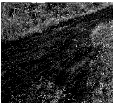
Organic soil makes a relatively poor trail tread because it maintains air spaces between particles that can become replaced with water. Hence this soil lacks bonding between particles, does not become solid when compacted, and holds a high amount of water when wet.
