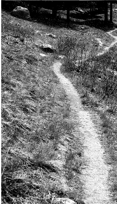
Limiting erosion. Limiting tread grades to short segments prevents major erosion by limiting the amount of water flowing down any segment. Each segment must drain to somewhere lower than itself. This is easiest when a trail traverses a slope.
