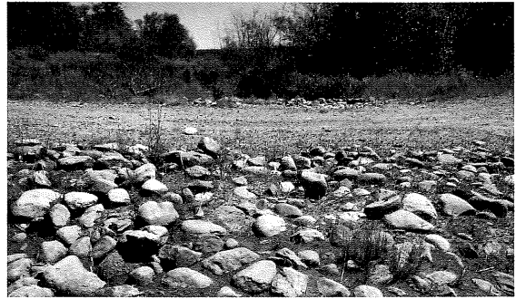
Overflow crossing with laterally stabilized aggregate. Geotextile and geocell were used on both the top and sides of this causeway to stabilize for flood flows in case culverts fail. The tread was capped with Class 5, but cobbles and soil were left exposed on both flanks. Note the dip, right, which concentrates low flows.
