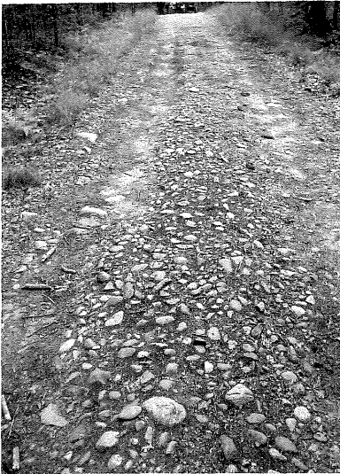
Pit run sand and 2- to 4-inch cobbles were used to harden this forest road segment with an approximately 10% grade. Although ATVs displace some of the smaller cobbles and gravels, larger particles – imbedded in sand and compacted – remain in place.
