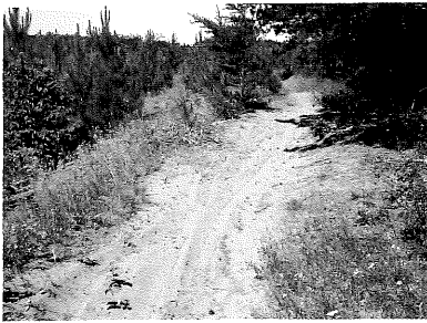
Round-grained "sugar sand" has zero cohesive strength and cannot hold any tread shape.
