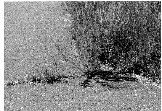
This trail, which is also only three or four years old, is showing the impact of prairie grasses and weeds growing in pavement cracks. Keeping the shoulder mowed and filling cracks each year is a reasonable and cost-effective solution here, rather than using a root barrier.
