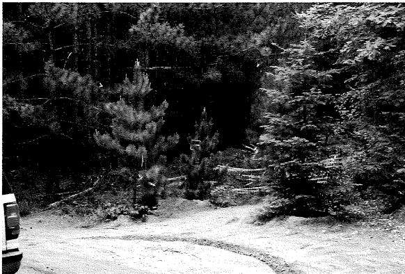
A straight forest road/trail was rerouted to the left (where the vehicle is heading) and the old route was hidden with a low berm (behind the orange fence) and planted conifers. The conifers largely hide the berm and the former route. This closure would have been even more successful if more trees had been planted and if the grade and ground cover in front of the berm were completely restored.
