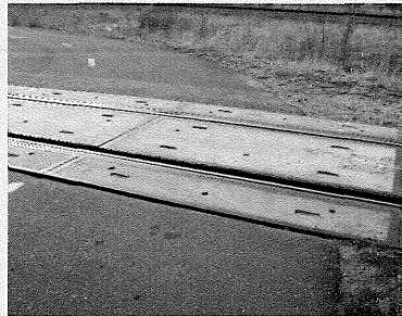
The concrete and steel framing of this crossing is very durable and stable. Although acceptable, the less-than-90-degree crossing angle increases the chance of catching a wheel.
