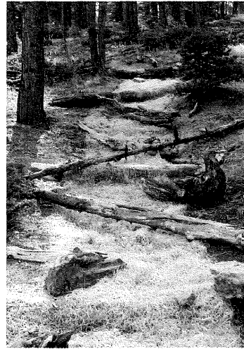
Stabilization of gullied fall-line trail with check dams made from dead trees (left) and with check dams plus erosion control blanket in steeper areas (right). Erosion control blanket doubles as mulch.
