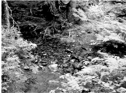
This dip on a hiking trail is strengthened by surrounding trees and vegetation. With a few rocks and rubble used to harden it, the dip is also the least muddy and most stable place to cross this intermittent drainage.
