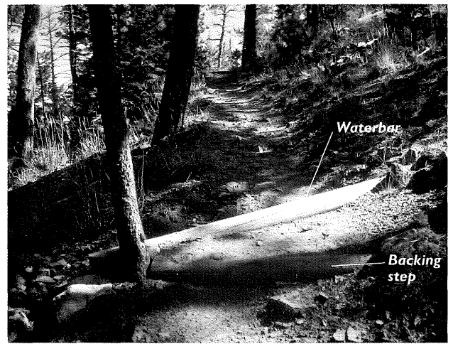
A backed waterbar is sometimes necessary on steeper tread grades. It also makes for a comfortable step in the ramp behind the bar while it stabilizes the ramp. This is typically built as a riser perpendicular to the tread. Note how this waterbar is anchored on the tree at left.
