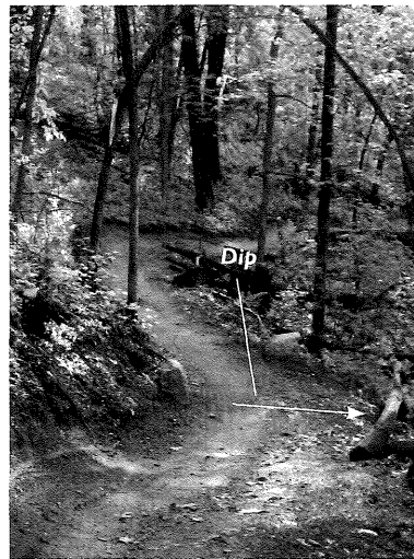
This dip on a hiking trail is strengthened by surrounding trees and vegetation. With a few rocks and rubble used to harden it, the dip is also the least muddy and most stable place to cross this intermittent drainage.
