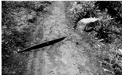
(Upper left) A 30 percent tread grade needs higher maintenance. The bar is silted in and partially collapsed on the outsloped tread for mountain bikes. The bar is also too short on the right side.
