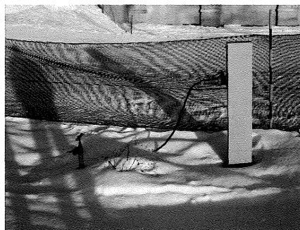
Water service and electrical pedestals are spaced along the trail at roughly 300-foot intervals. This makes the length of hose and electrical cord from the machines less cumbersome. Water is supplied from a pond or high-capacity well.
