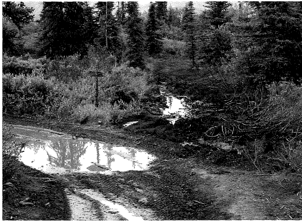
Problem: Bypassing causing unacceptable ecological impacts. Immediate closure of the trail will be necessary to curtail this from getting worse. The area is simply not well suited for an ATV trail.
