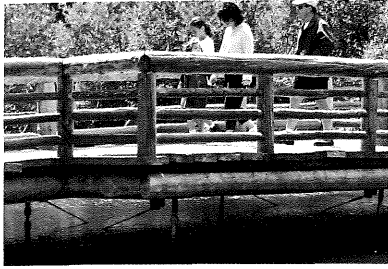
Four helical screw piles support the center of this bridge. The piles are under a widened deck section that encourages visitors to pause on the bridge. Cross-bracing prevents side-to-side swaying.
