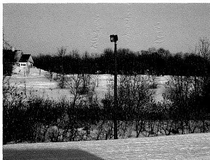
The common pole-mounted high-pressure sodium fixture faces down the trail in the direction of travel to avoid putting light in the face of the skier and night ski. With buried wire, a natural-colored pole, and a small fixture, the light serves its purpose with minimal visual intrusion.
