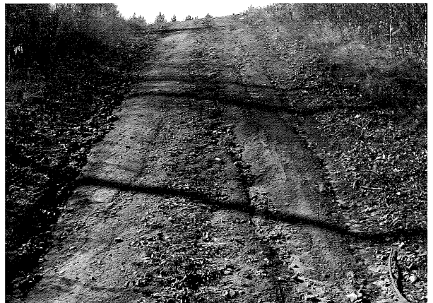
Problem: Erosion due to fall-line alignment. In both of these cases, the trail follows the fall line (i.e., is aligned straight up the slope), creating an opportunity for erosion. In the left photo, erosion is becoming a problem and soil is migrating to the base of the slope. If periodically maintained, this trail could remain reasonably stable, although a better solution is to realign it. In the right photo, erosion of a forest access route is clearly becoming an issue with increasing use and exposure to the elements. Realignment or closure of this segment will ultimately be necessary to keep this trail sustainable.
