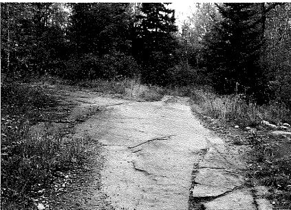
A naturally hardened crest offers an interesting anchor to this ATV trail. The rock outcrop is also very stable, which allows for a steeper approach.
