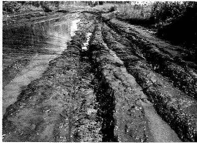
These deep and spreading mud tracks on this ATV trail represent a clear case where tread hardening (or rerouting) is needed. The lack of physical barriers to keep the trail to a desired width is also evident in this photo.
