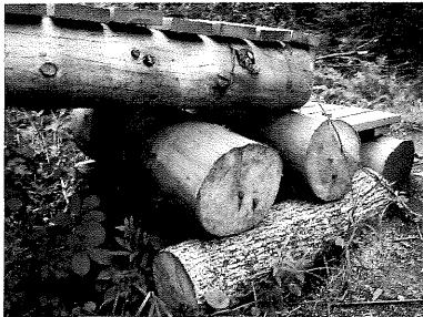
This small cribbed foundation is designed to be rustic and low impact. Logs are nailed together and rest directly on undisturbed ground.
