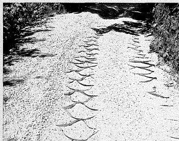
On this ATV trail, the crushed limestone cap layer used is too lightweight and too small in particle size to withstand displacement. While the stiff geocell webbing will prevent further deepening, it will need to be top dressed with replacement limestone every year.
