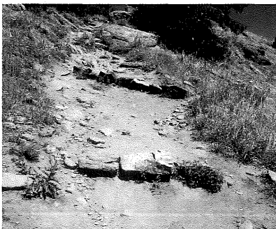
Visitor bypass. Some hikers perceive these rough stone waterbars as obstacles and bypass them. Note how new treads are forming on both sides of the waterbars.
