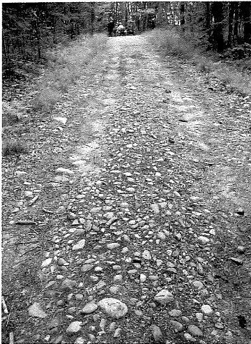
These natural rock cobbles form a stable ATV trail tread on this fall line downslope that has withstood years of use. Its sustainability is due to considerations of many of the factors listed on the previous table.
