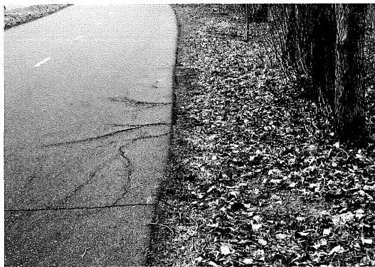
This trail, which is only three or four years old, is showing the impact of shallow-rooted trees on the trail pavement. Left unchecked, this segment will continue to degrade and become rougher to ride on. A root barrier would be reasonable in this situation.
