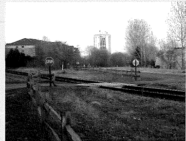
Although smooth, this crossing is only as wide as the trail. Given the abruptness of the crossing, more width would make the turn more comfortable and increase the margin of safety.
