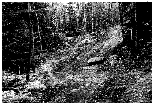
(Right) Rolling grade is used on this OHV trail to drain the tread, control erosion, and create challenges for ORV drivers. The tread is intentionally rough and extreme — yet erosion is limited by very short tread watersheds.
