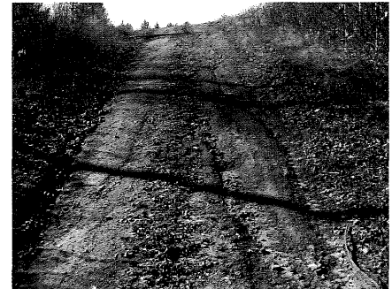
The lack of ground cover on this steeper hill is allowing erosion to take hold, making the trail unsustainable for summer use and increasingly rough for winter use.
