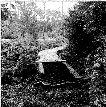
Geocell over wet organic soils. Behind the staked board, the cells have already been filled with crusher fines and compacted. This is 4" thick geocell installed in a turnpike, but the wood sides serve mostly to hide the edges of the raised geocell webbing. Although not used here, geotextile should be used under the geocell to help prevent cell fill from mixing with unstable soil below.
