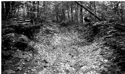
Fall line alignment, entrenched tread. This former ice road is up to 5 feet deep. Although it does not appear to be actively eroding, it eroded once and could again. The existing fall-line trench cannot be drained and should be avoided as a trail.
