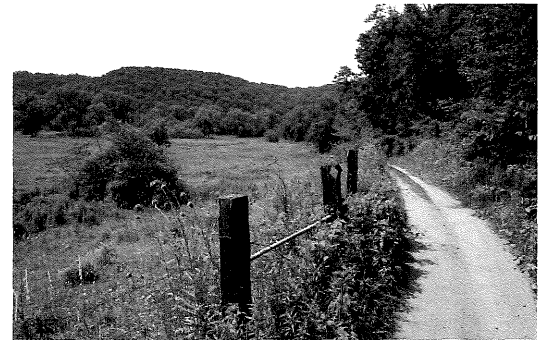
Sideslope alignment on abandoned township road. Following the lower edge of the slope at right while staying above the nearly level grassland below, this portion of the Southeast Minnesota ATV Trail is both sustainable and enjoyable.
