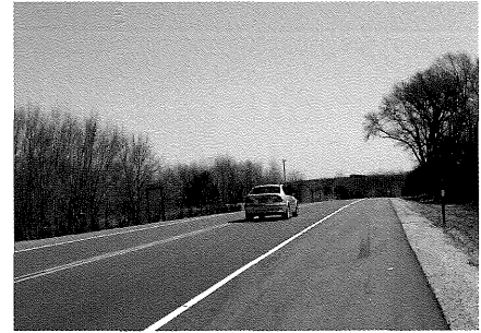
Bike route on wider, higher speed roadway. Once speeds get above 50 mph, a minimum 6 foot shoulder is recommended to provide reasonable separation between bicyclists and motor vehicles.
