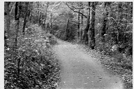
Winding up the grade. By traversing up a steeper grade with modest switchbacks and landings, this trail is less imposing (and more fun) than it might otherwise be if the trail climb were more direct.
