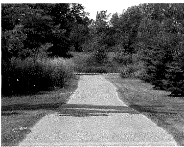
The design speed for a neighborhood trail such as this is lower than that for a regional or state trail. Most often, trail users will travel in the 8- to 15-mph range on a bicycle, a more leisurely 2- or 3-mph on foot.
