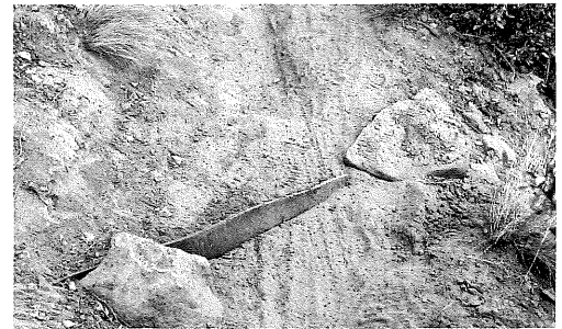
(Upper left) A 30 percent tread grade needs higher maintenance. The bar is silted in and partially collapsed on the outsloped tread for mountain bikes. The bar is also too short on the right side.
