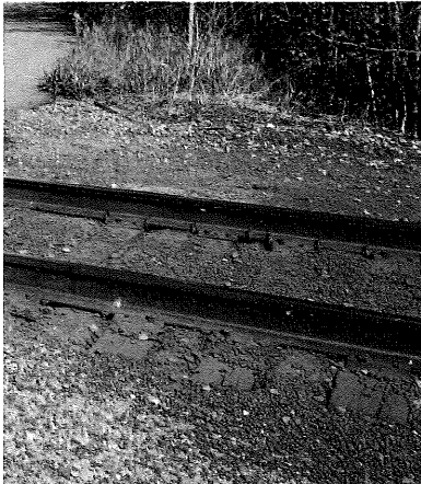
Once ties and steel tracks are removed from a typical railroad grade, the remaining ballast is uneven and too coarse for placement of trail pavements. Typically, the subgrade is prepared using a rotary soil mixer that mixes the top 16 inches into a well-graded subgrade mixture.
