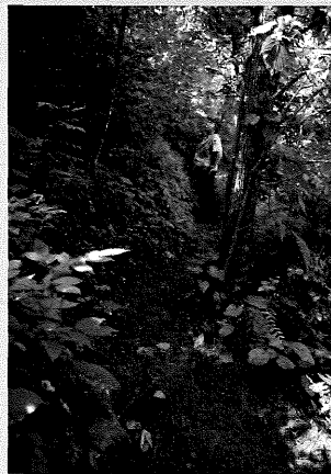
Jogging, near-level. The trail jogs up above a tree to create a crest. The tree anchors the crest and its roots help resist crest displacement. Note the very steep sideslope. (Horse trail)
