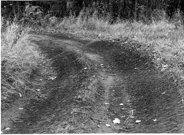
Superelevated corners can be very sustainable if they stay within the established treadway. However, if trail "creep" begins to occur, the trail starts to slide into an unsustainable condition.
