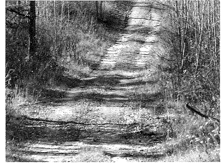
Low-flow crossing. This crossing only occasionally flows during heavy rains and dries up quickly thereafter, requiring no hardening to keep it sustainable.
