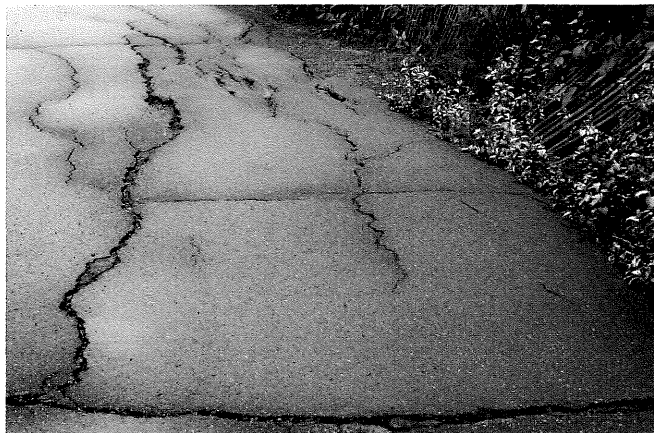
Both of these trails have 2 inches of asphalt over a 4-inch aggregate base. As shown, both are structurally failing. Because they weren't built with adequate structural integrity to begin with, each will have to be completely replaced well before the end of a typical design life of 15 or more years.
