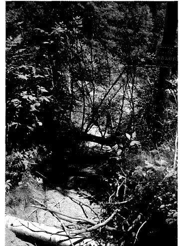
This deeply eroded horse trail in sandy soil was closed with slash and a trail closure sign pending further action. Further erosion could be reduced by adding considerably more thick slash.
