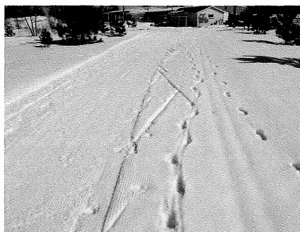
Grooming underway on this trail, with the left side packed under the first pass. Grooming technique is as much art as science, and "time on the machine" is the best training.
