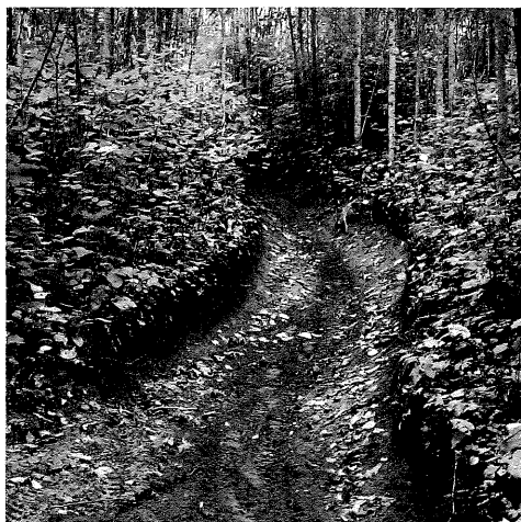
This five-foot-wide sandy tread is eroded up to 30 inches deep. Subsequent trail use displaces more soil that quickly smooths over the ruts. This smoothing can disguise the severity of erosion, making it seem as if the problem is not as bad as it actually is.
