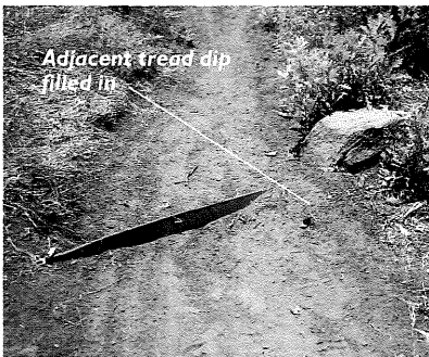
Sedimentation. This flexible waterbar is no longer functional because of sedimentation, which allows water to now flow over the top of it.
