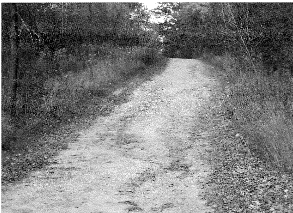
Problem: Erosion due to fall-line alignment. In both of these cases, the trail follows the fall line (i.e., is aligned straight up the slope), creating an opportunity for erosion. In the left photo, erosion is becoming a problem and soil is migrating to the base of the slope. If periodically maintained, this trail could remain reasonably stable, although a better solution is to realign it. In the right photo, erosion of a forest access route is clearly becoming an issue with increasing use and exposure to the elements. Realignment or closure of this segment will ultimately be necessary to keep this trail sustainable.
