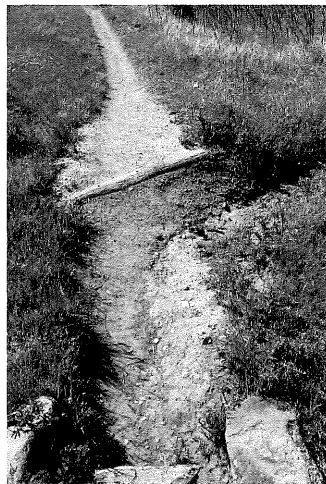
Timber is used to reinforce the top of a filled crest. Note that water is smoothly diverted into the well-formed outlet without touching the timber.
