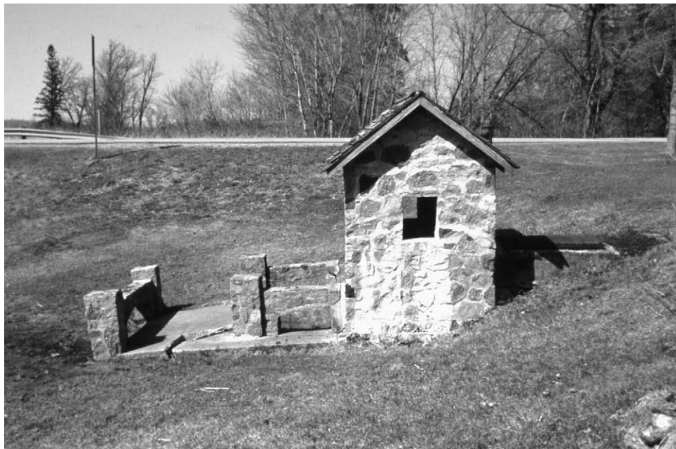
Fig 2. Spring enclosure, Hewitt Roadside Parking Area, April 2003.
