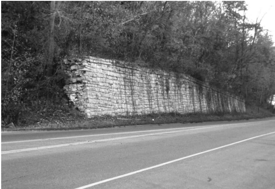
Fig. 8. Stillwater Retaining Wall, Nov. 2002.
