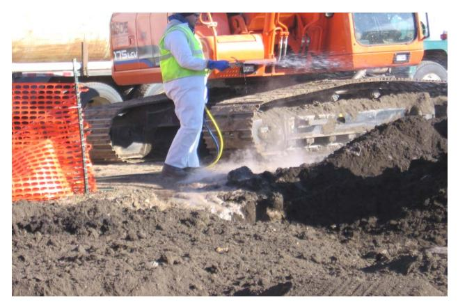
Carbon Carbon double bonds break as PCP begins to mineralize:
