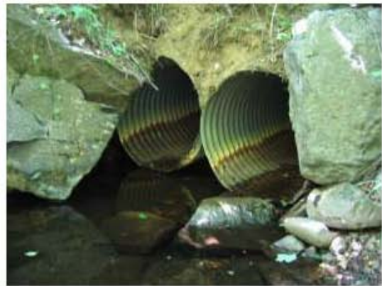
A double culvert along the NSST, installed in 1982, that needs replacement. These culverts are too short for the current width of the trail and were improperly placed.
