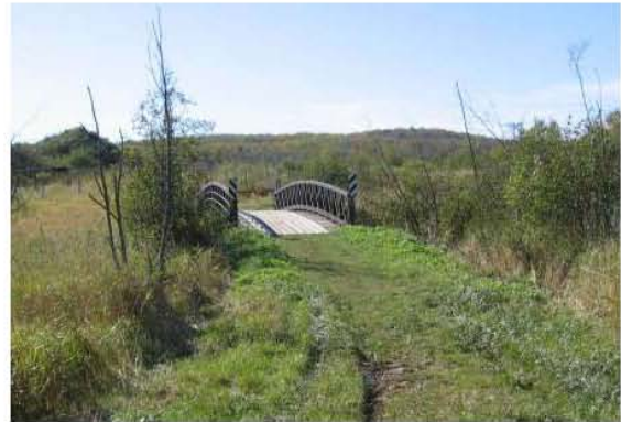
NSST crossing over East Branch Amity Creek, a Designated Trout Stream and impaired water downstream of the trail, St. Louis County.
