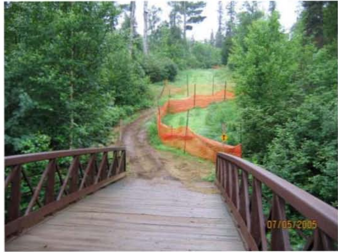
An existing hill reroute on the portion of NSST open to ATV use. The orange snow fence is used to direct ATV traffic across the snowmobile trail route, which is along the fall line (hill grade is 23%). The bridge is located over the West Branch Baptism River.
