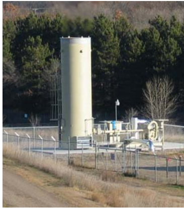
Photo 5: Gas flare at the Anoka-Ramsey Landfill
