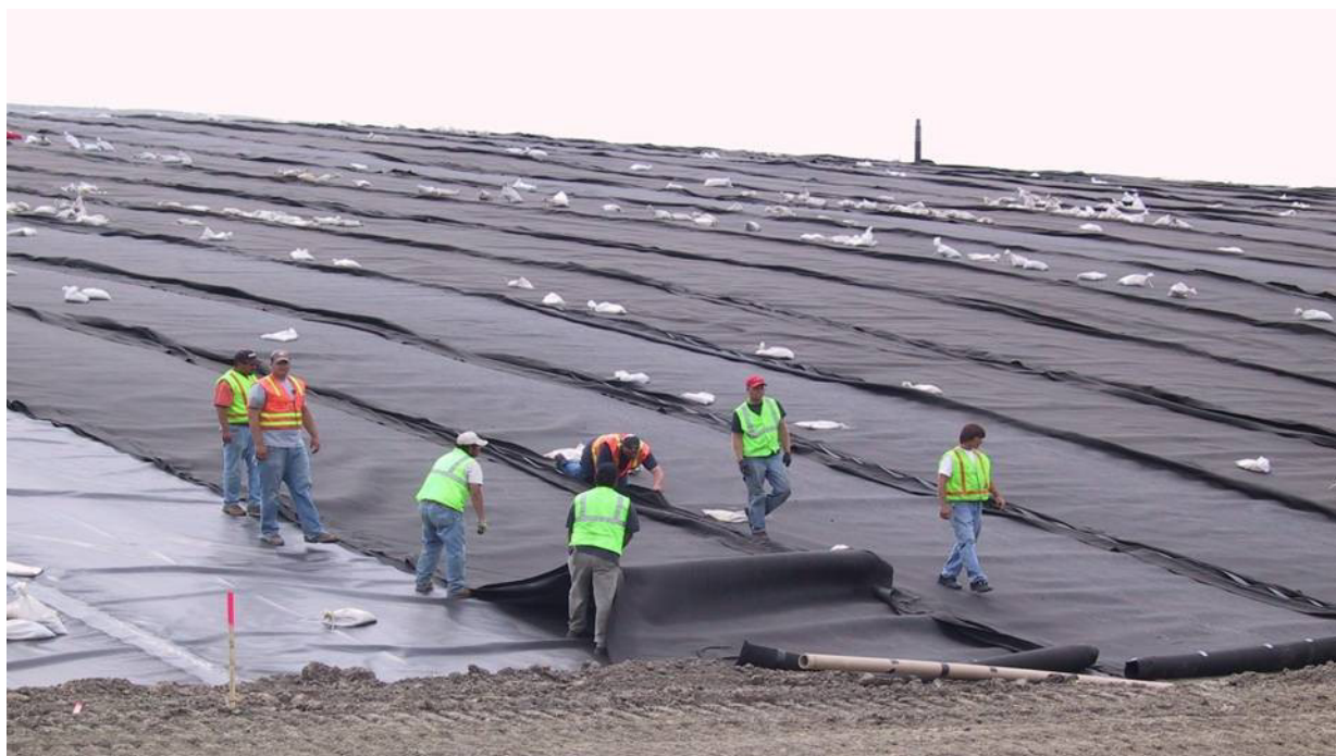
Photo 2: Liner installation at the East Bethel Landfill, 2006
