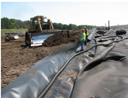
Photo 3: Construction of Toe Drain at the East Bethel Landfill, 2006
