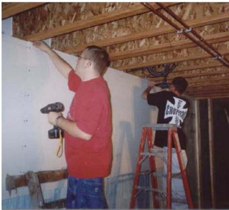
Jeremy Meis and Nick Neal installing sheet rock.
