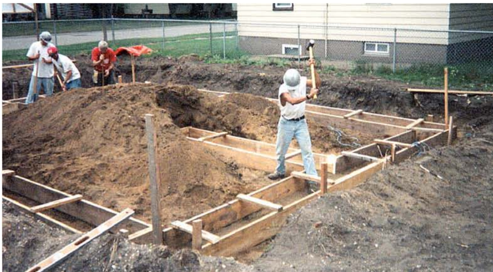
Youthbuilders set footings for a concrete foundation.
