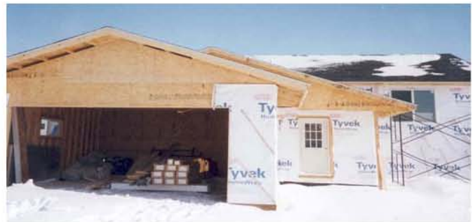
Stress panel house built by CEP Youthbuilders.
