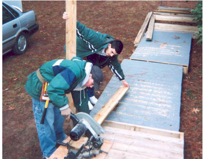
Brett Gremminger and Jon Wilson saw boards while building a wheelchair ramp for an elderly homeowner.
