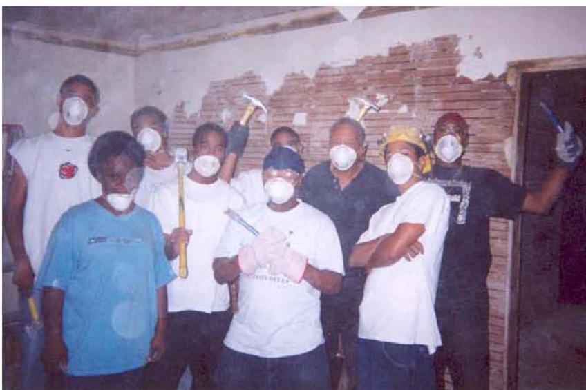
Summit Youthbuilders renovating a home in Minneapolis.
