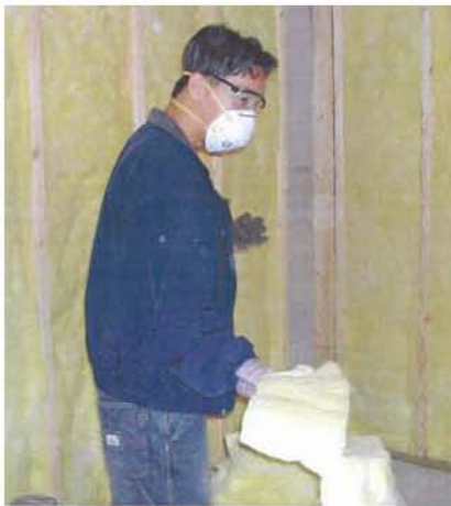
Dao Lee insulating the interior of a basement.
