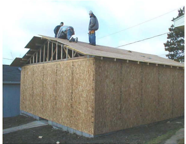
Above: Youthbuilders Ben Meyer, Chris Harfield, and Chris Stella finishing roof sheathing on a garage. Below: Exterior view of the Finnish Boarding House at Ironworld in Chisholm.
