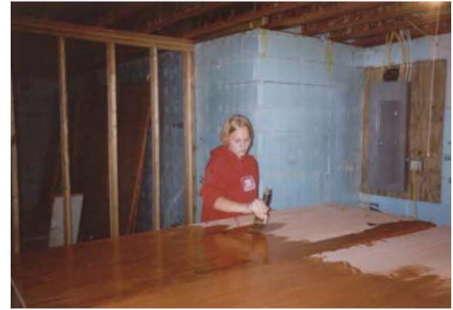
Ferrin Synhorst staining wood doors.
