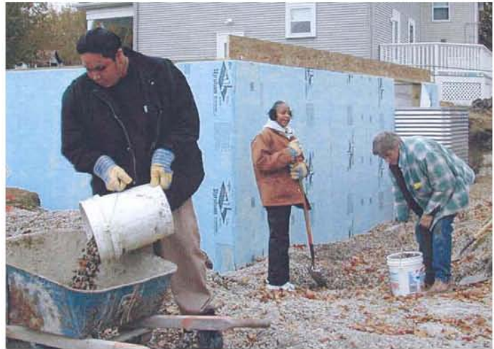
Raymond Johnson and Kentara Dean, with instructor Grant English, drain tiling around a south Minneapolis home.
