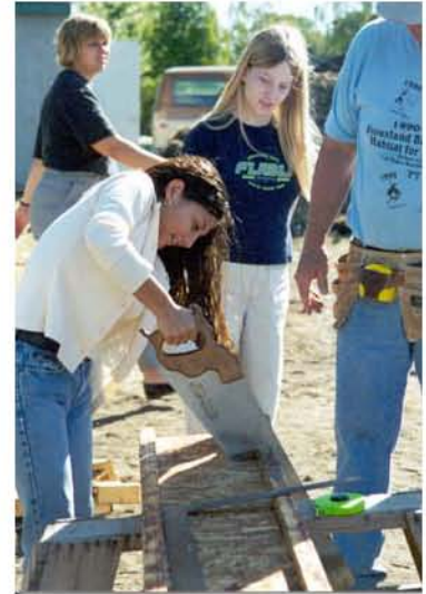
Willmar Youthbuilders constructing picnic tables for local park.
