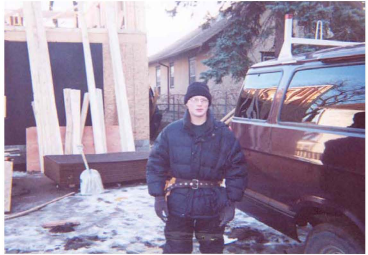
Nick Whaley prepares for a cold day of working outside on framing a house.
