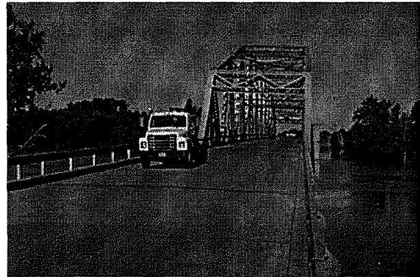
Above: This bridge at Drayton/Robbin will be replaced with a new 4,000 foot bridge in 2009. Construction cost estimated at $31 million.
