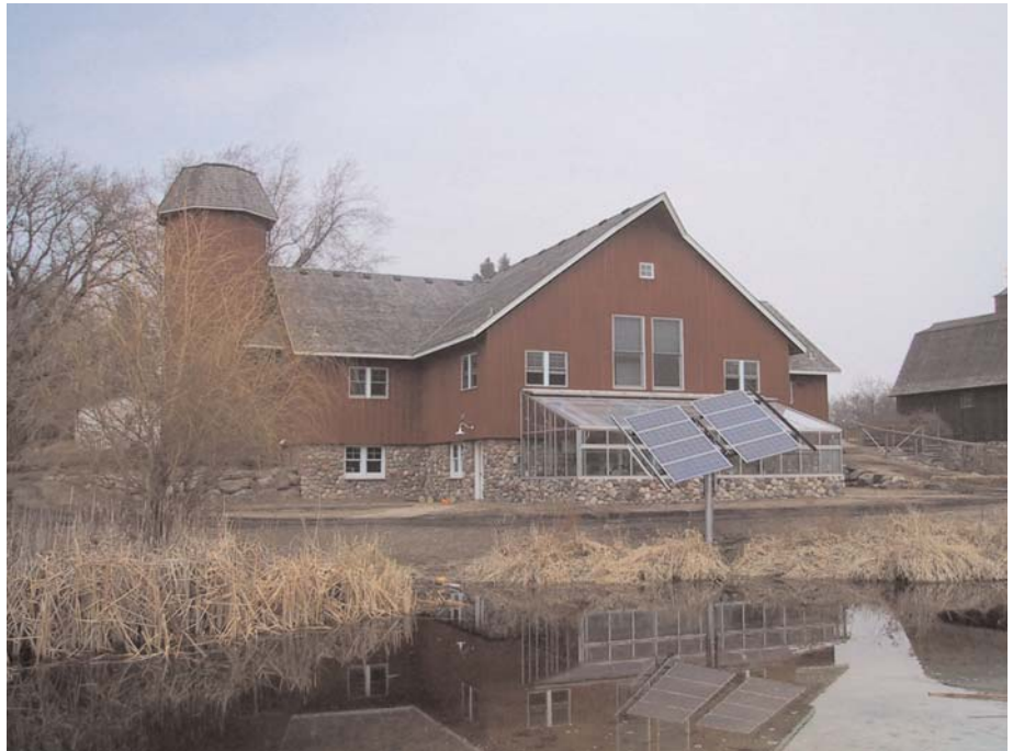
1 kW met metered dual axis tracking solar system located at Dodge Nature Center, West St. Paul, MN (Source: Dodge Nature Center)
