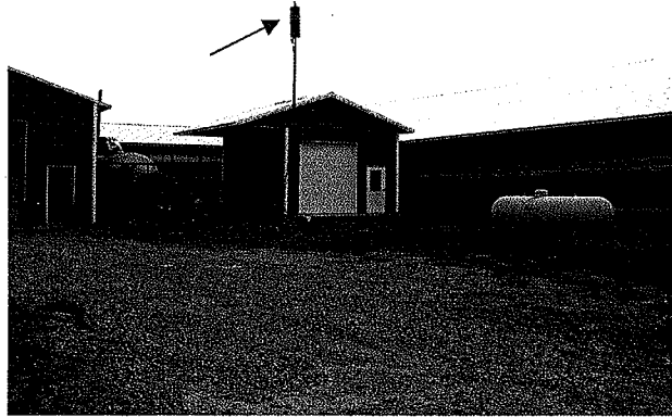
Water Tower next to Building
