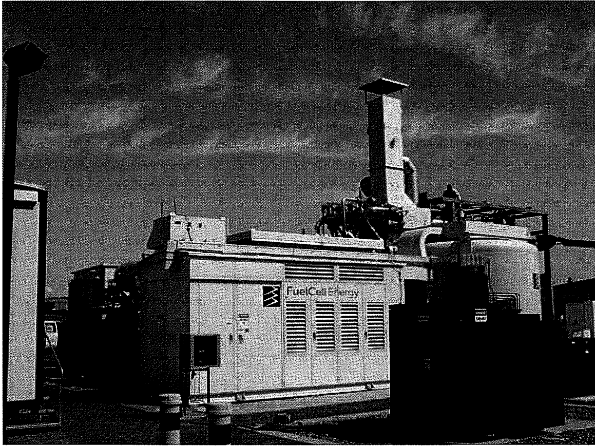
Molten Carbonate Fuel Cell, 1 megawatt, Fuel Cell Energy Inc. Danbury CN
