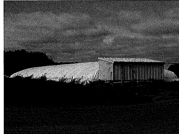
Anaerobic Manure Digester
