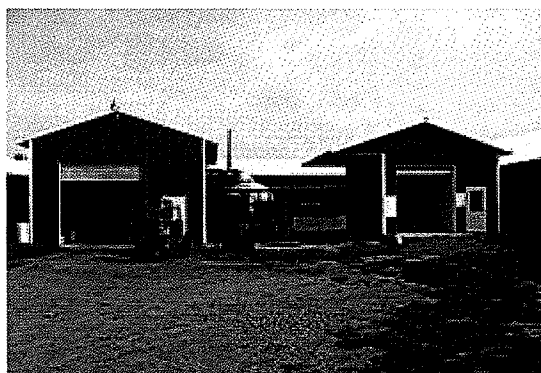
Existing engine generator building on left, alternative generation research building on the right housing 5kW fuel cell.
