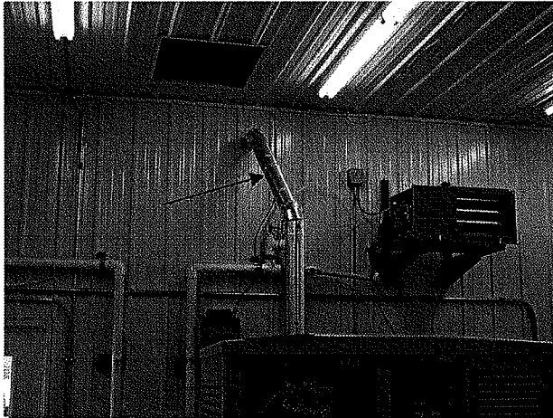
Vent for Fuel Cell Emissions
