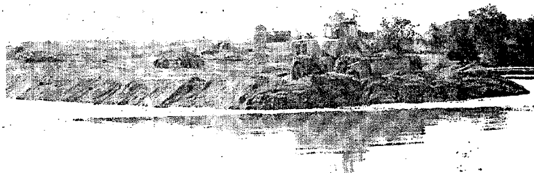
Fill placement for the Lake Lakota crossing. Total fill to across the lake was over 330,000 yards.
