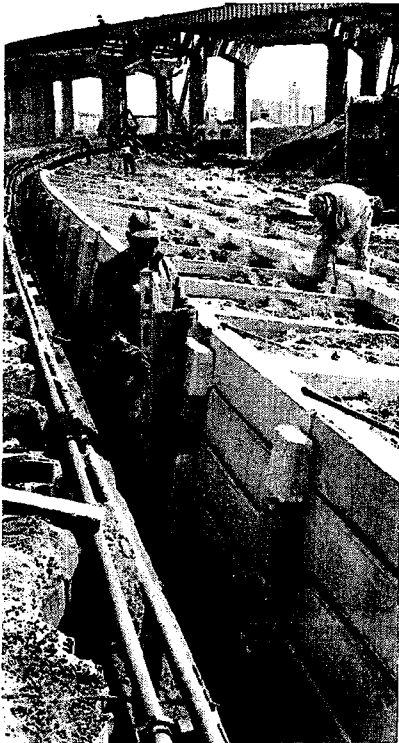
Details of cribwall construction along the Garfield Ave. northbound roadway are visible here. Alignment of units is under way. Note bridge in background.
