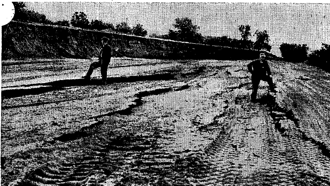
This view, looking south, of the slide which occurred at the Minnesota river bridge approach on Interstate Route 394 in Bloomington shows the main failure plane in the background, with some of the "companion" cracking in the foreground.
