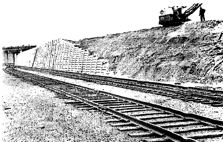
Shown here is the building of a cribwall supporting the reconstructed northbound roadway of Garfield Ave., adjacent to I.R. 535.
