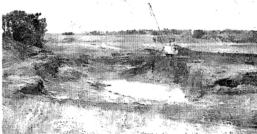
Swamp excavation for I 94 south of Evansville. The swamp cut at this location is 25 feet in depth and is part of more than one million yards swamp removal on the project.
