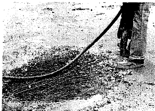
Potholes on the Hennepin Avenue ramp of I-94 in Minneapolis are repaired by maintenance workers from the Golden Valley district. The freeway will continue to require constant maintenance until its reconstruction is completed.
