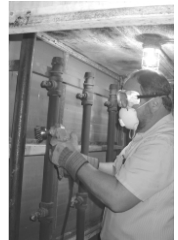
A St. Paul College staff member works to maintain the college's air handling unit.
