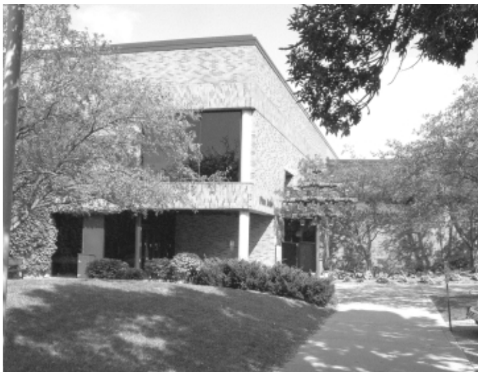
Renovation and an addition to the Fine Arts Building will add much-needed classrooms and labs.
