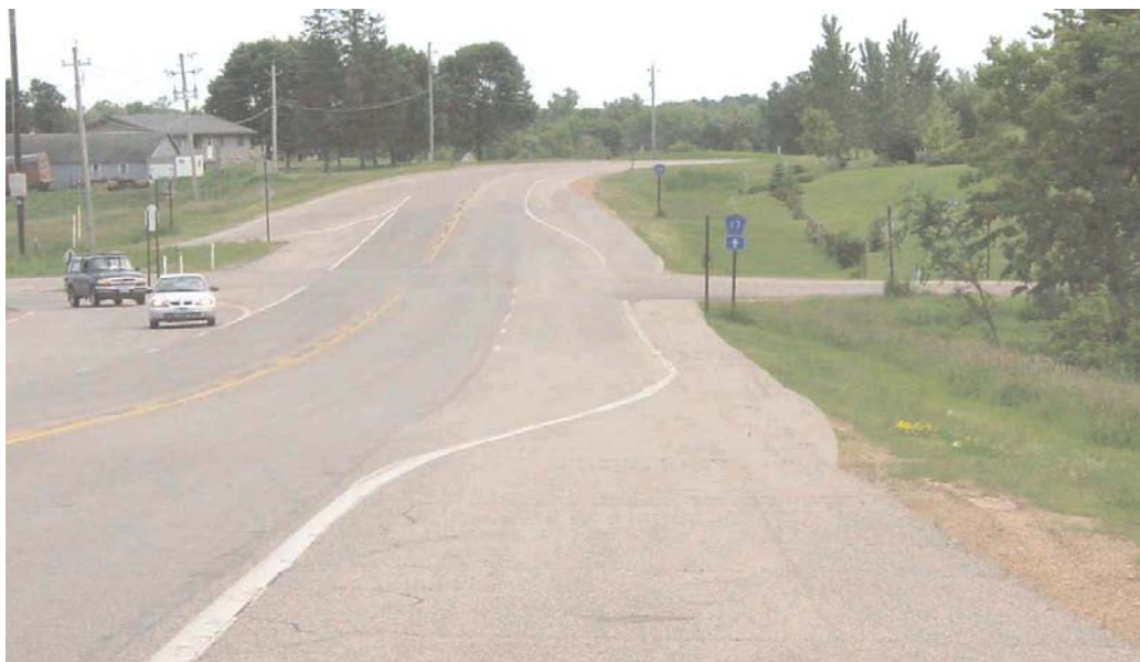
Figure 6: A small amount of extra asphalt adds a thoughtful measure of safety for cyclists using the shoulder
