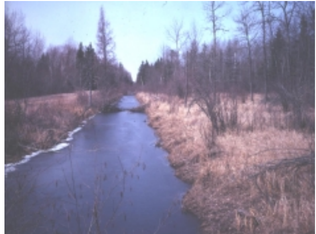
Figure 10 – Example of Drainage Ditch in Northern Minnesota
