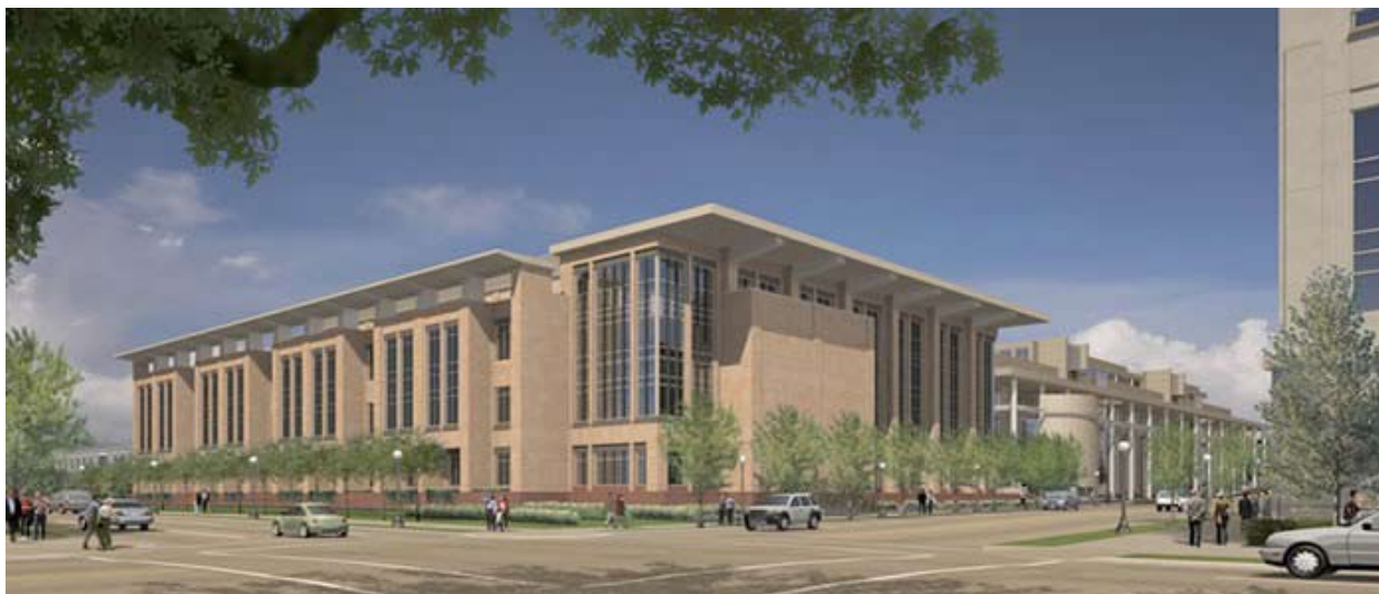
Public Health/Agriculture Laboratory building at 601 North Robert Street
