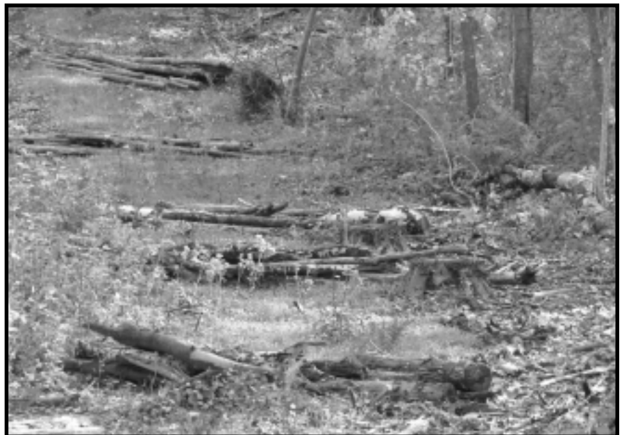
Slash water bars are installed to divert the volume, velocity, and direction of water flow, thus reducing the amount of sediment eroding on the skid trail. Photo by Mike Phillips/Minnesota Forest Resources Council
