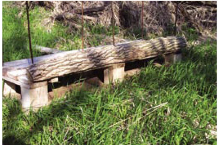
Constructed “lunker” structure used to create overhead bank cover for trout.
