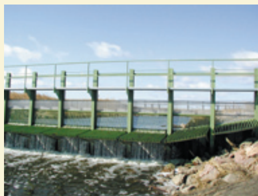
A MECHANICAL FISH BARRIER CONSTRUCTED BY THE MINNESOTA DNR AND DUCKS UNLIMITED ON U.S. FISH AND WILDLIFE SERVICE LAND DOWNSTREAM OF THE WATER CONTROL STRUCTURE IN 2003 PRECLUDES FISH FROM RE-ENTERING BIG SLOUGH.
