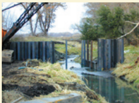
PRIOR TO TREATING LAKE CHRISTINA WITH ROTENONE IN 2003, THREE NEW WATER CONTROL STRUCTURES AND TWO MORE FISH BARRIERS WERE CONSTRUCTED ON WATERWAYS FLOWING INTO THE LAKE. BECAUSE UNIQUE CIRCUMSTANCES PREVENT THE LAKE LEVEL FROM BEING MANAGED VIA DRAWDOWNS, THE INLET STRUCTURES ARE BEING UTILIZED TO MANAGE THE AMOUNT OF WATER ENTERING THE LAKE AT STRATEGIC TIMES.
