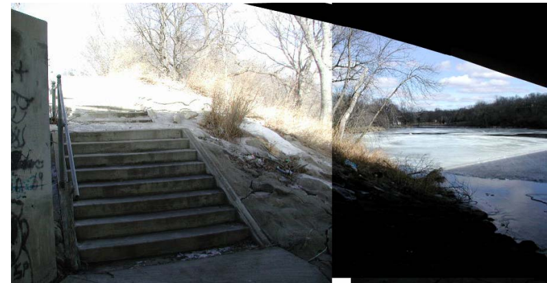
HWY. 212 BRIDGE UNDERPASS TRAIL
