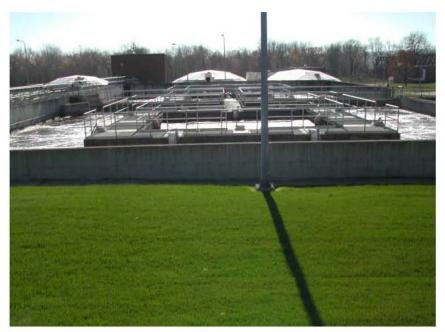
Figure 5.1.3.2 - Aeration Tank, New Ulm WWTF
