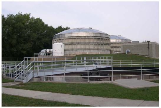
Figure 5.6.1.2 - View of Covered Plastic Media Trickling Filters, Faribault WWTF
