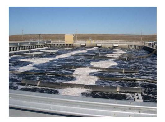
Figure 5.4.1.2 - Photograph of the Mixed-bed Suspended Media Nitrification System, Moorhead WWTF
