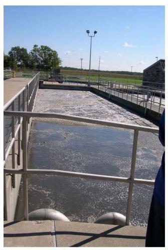
Figure 5.2.1.3 – Aeration Tank Showing Initial Unaerated Anaerobic Contact Zone St. Cloud WWTF
