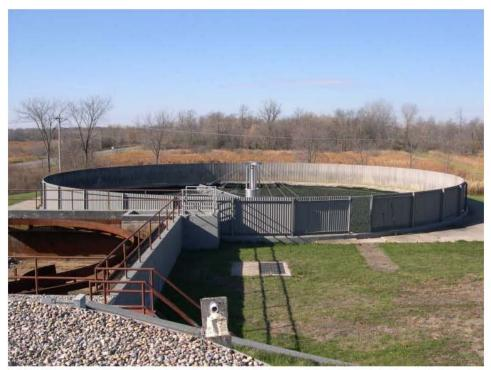
Figure 5.5.1.2 - Trickling Filter, Detroit Lakes WWTF
