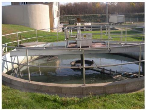
Figure 5.6.4.3 - Gravity Thickener, Little Falls WWTF
