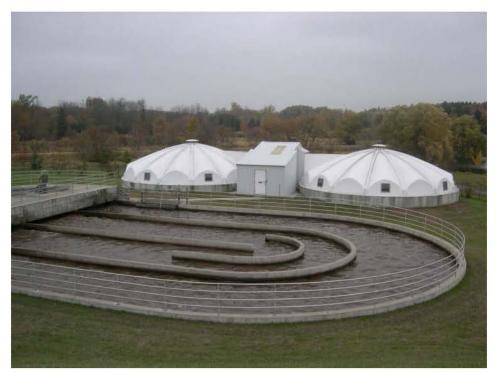
Figure 5.3.1.2 - Oxidation Ditch, Wadena WWTF
