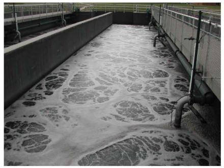
Figure 5.6.2.3 - Aeration Tank, Marshall WWTF
