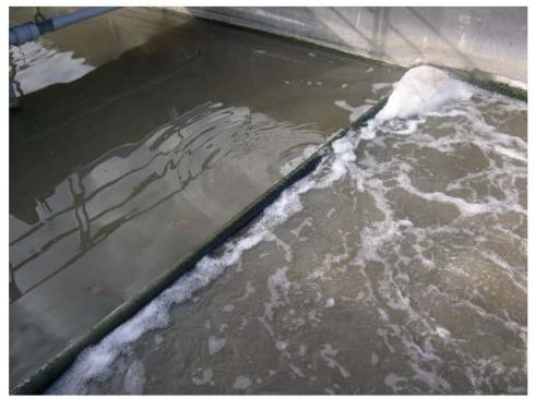
Figure 5.2.2.3 - Anaerobic and Aerobic Zones, Fergus Falls WWTP
