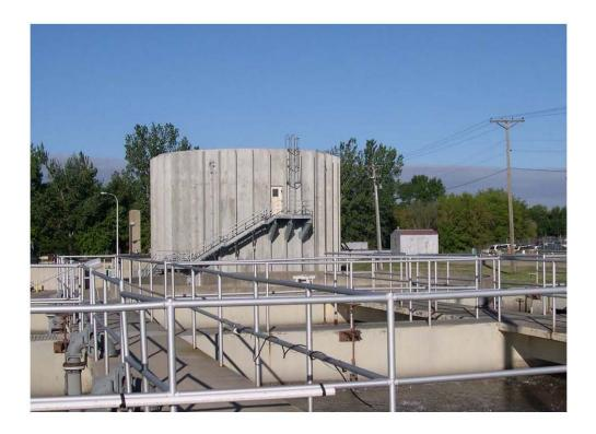
Figure 5.6.3.2 - View of Plastic Media Trickling Filter and Aeration Tanks, Glencoe WWTF
