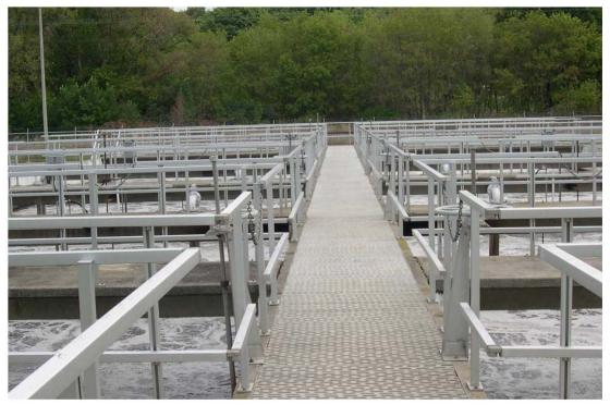
Figure 5.6.1.3 - View of Two Parallel Aeration Tanks, Faribault WWTF
