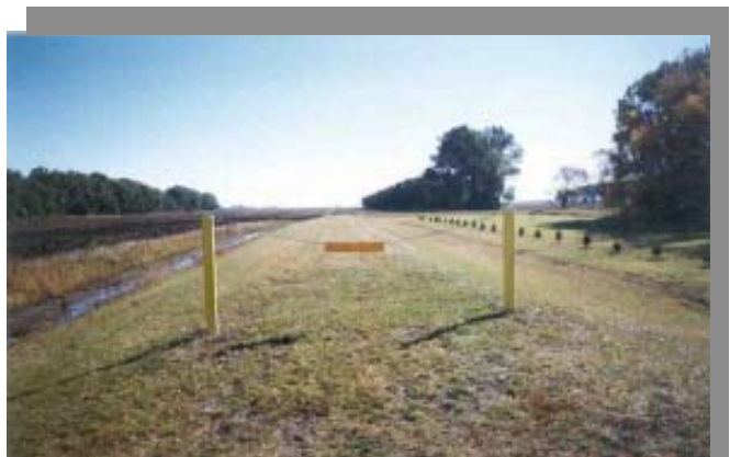
A small levee now protects Orchard Estates
