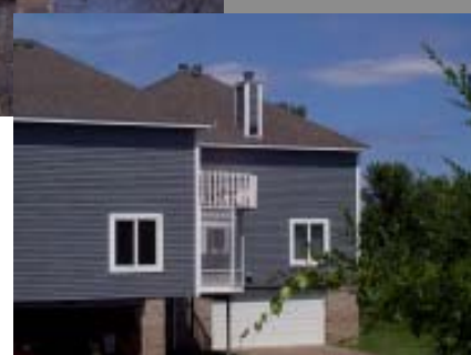
Townhouse with tuck-under garage that opens during the flood
