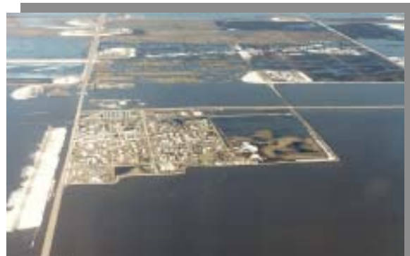
Levees protected Perley in 1997
