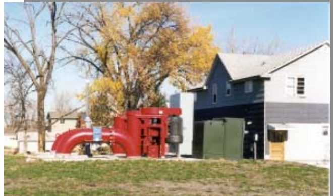
New pump to keep the city of Breckenridge dry
