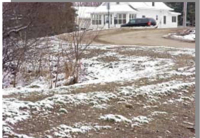
A small levee protects homes in the town of Dayton, at the confluence of the Crow and Mississippi Rivers
