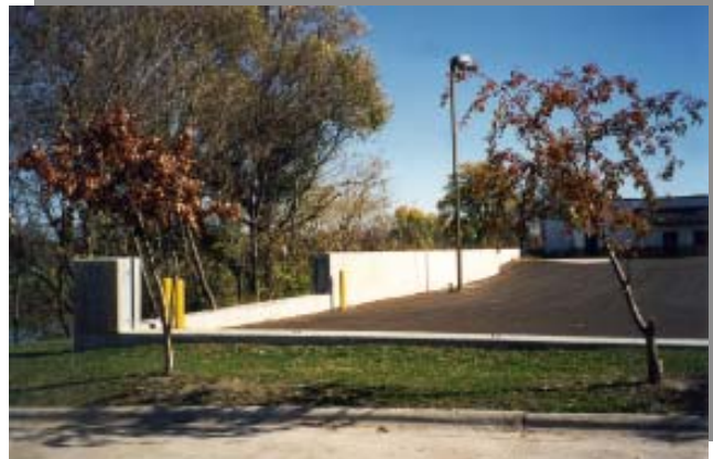
A small invisible floodwall protects downtown Breckenridge
