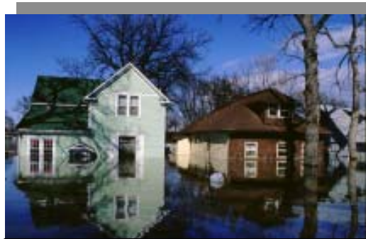
Every home in the Sherlock Park neighborhood was flooded
