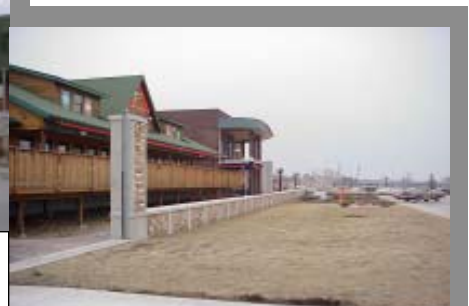
Floodwall in place
