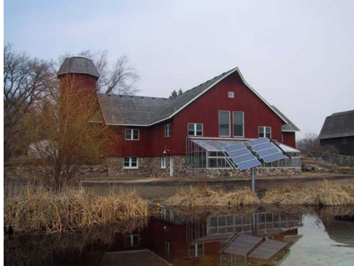
1 kW met metered dual axis tracking solar system located at Dodge Nature Center, West St. Paul, MN Source: Dodge Nature Center
