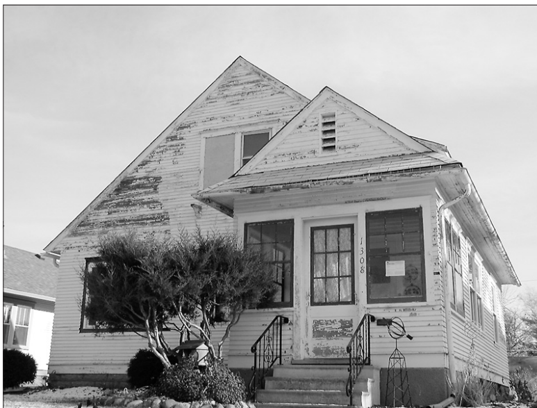
Most cities' property maintenance codes address the condition of exterior surfaces.
