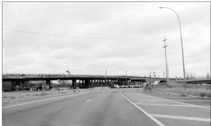
The Department of Transportation was asked to file a 16C violation memo for work related to the light rail transit project.
