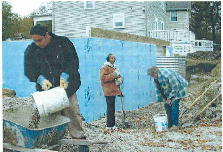
Raymond Johnson and Kentara Dean, with instructor Grant English, drain tiling around a south Minneapolis home.
