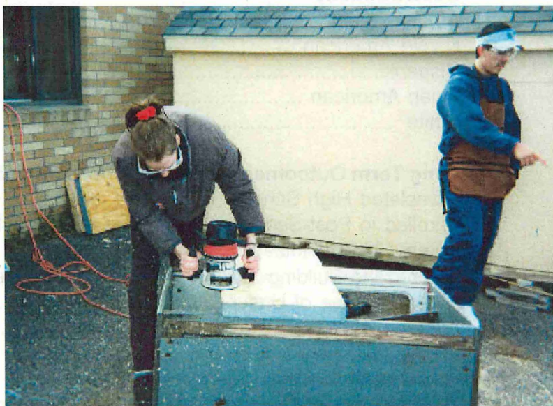
Wabasha Youthbuilder, Amy LaFond, works hard on the job.
