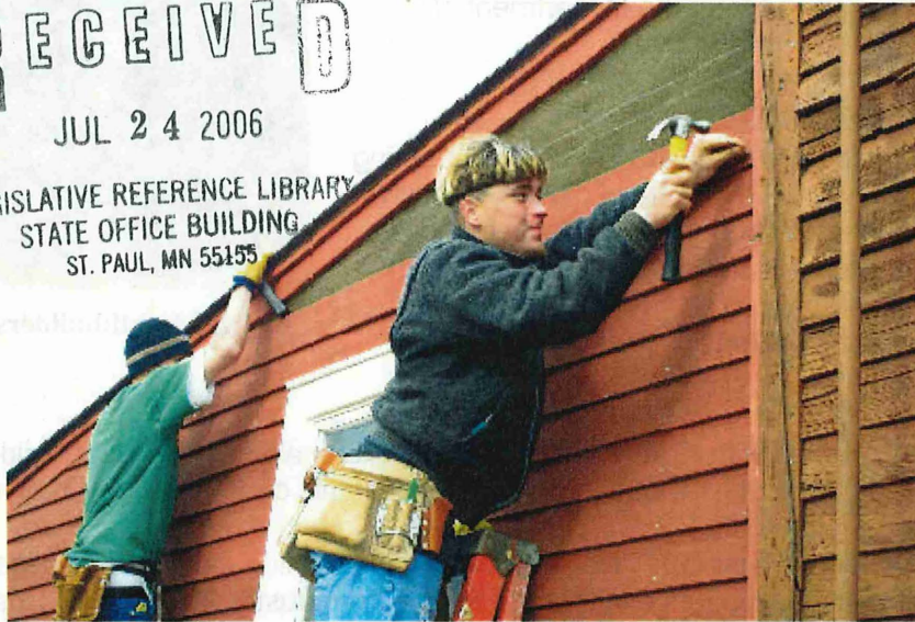
AEOA Youthbuilders, Josh Locke and Matt Gaige, siding the Finnish Boarding House, Ironworld, Chisholm
