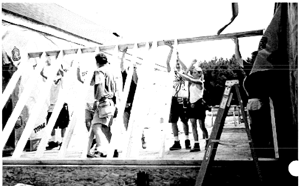
CSEC Youthbuilders framing a child care facility
