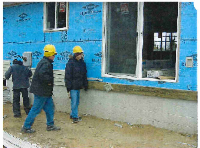
Bi-CAP Youthbuilders insulating exterior walls
