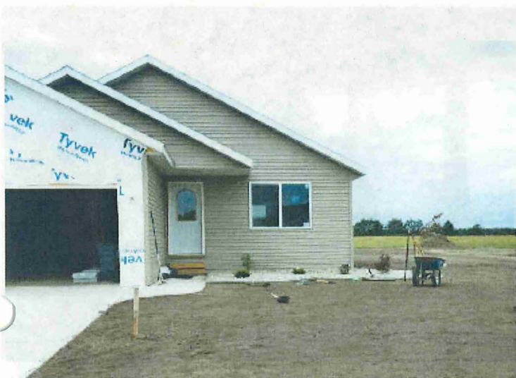
Stress panel house built by Youthbuilders in 2002 (various stages of construction)
