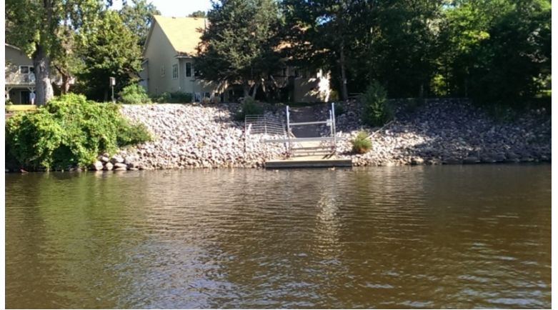
Figure 12. Example of riprap installation extent greater than needed to control erosion, with significant impacts on riparian vegetation and habitat.
