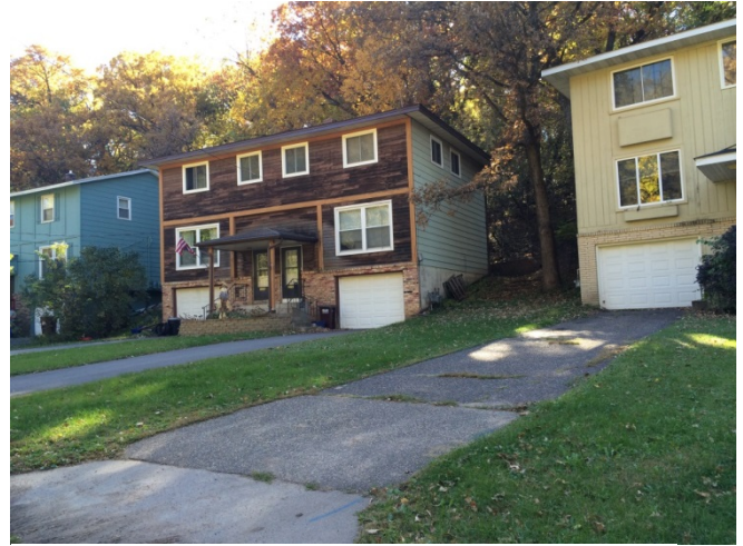
Figure 8: Existing structures near bottom of bluff under proposed bluff definition.
