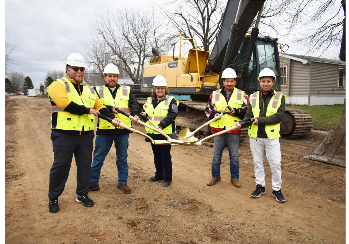
Members of Sungold Heights Cooperative in Worthington, MN celebrate the groundbreaking of their water, sewer, and road rehab project in 2021.
