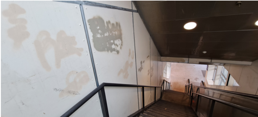
Figure 12: Lake St/Midtown Station Interior After Anti-Graffiti Wallpaper Installed
