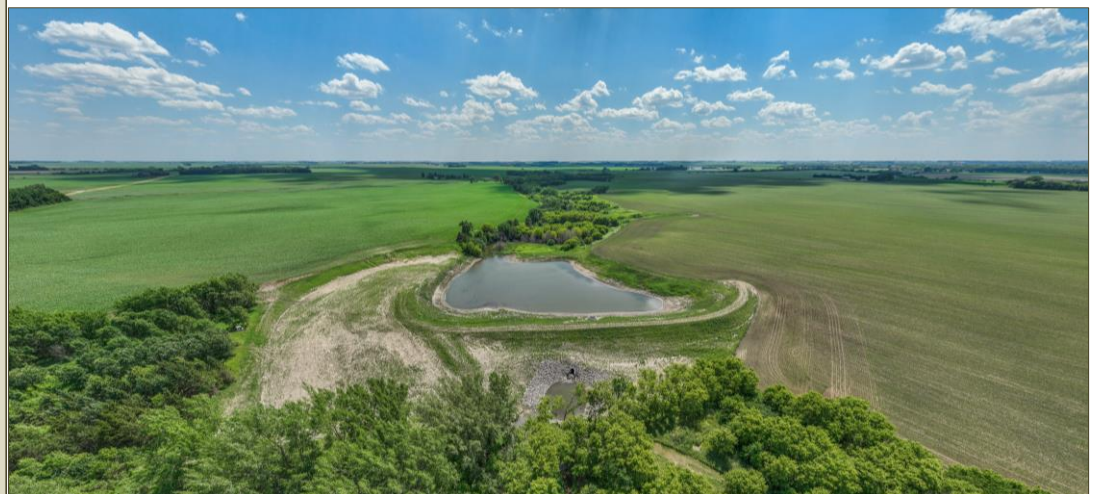
SPRINGDALE 19 GRADE STABILIZATION (Redwood County, 2021)
