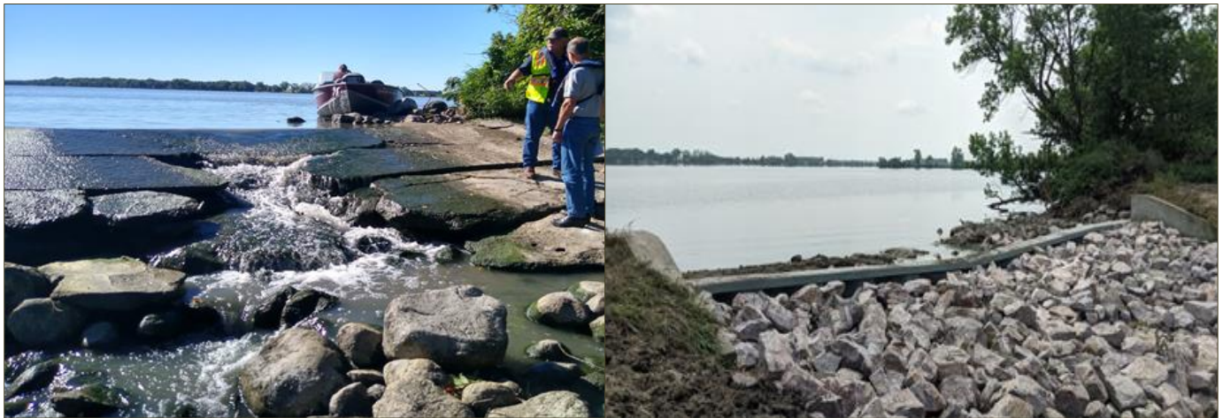
LAKE BENTON OUTLET RESTORATION (Lincoln County, 2021)
