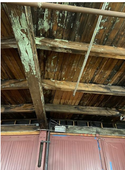
Compromised ceiling due to leaky roof
