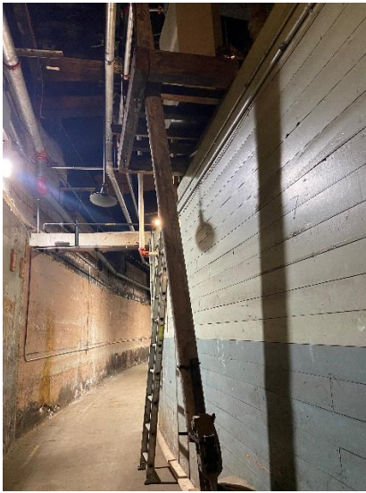
Posts supporting cracked beams
