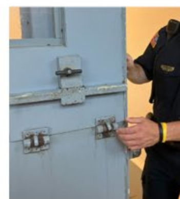
Rusting manual locks on cells
