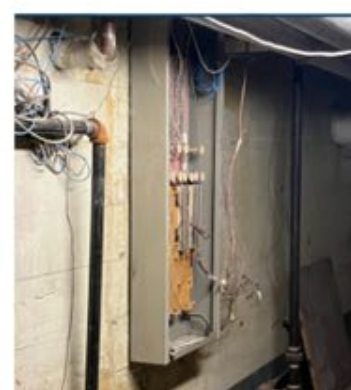
Exposed and outdated electrical wiring
