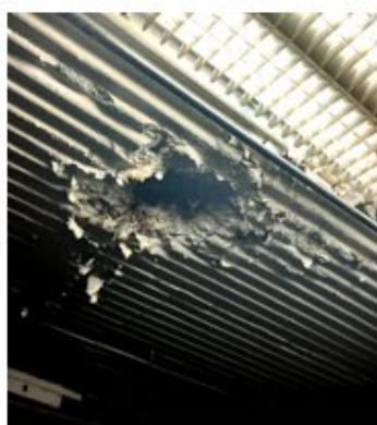
Hole in ceiling that is continuously growing
