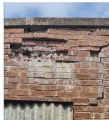
Crumbling brick in outside walls
