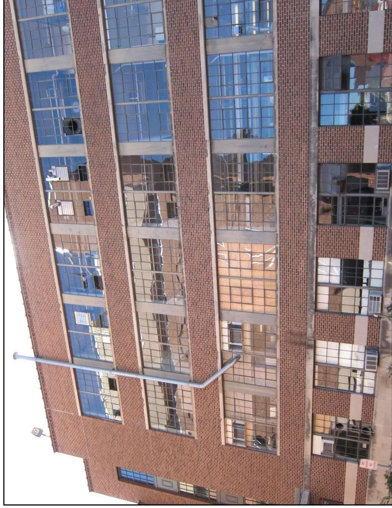
Left: Mechanical Engineering Building; improvised HVAC piping, window A/C units, and makeshift window coverings Right: Typical ab interior pre-renovation
