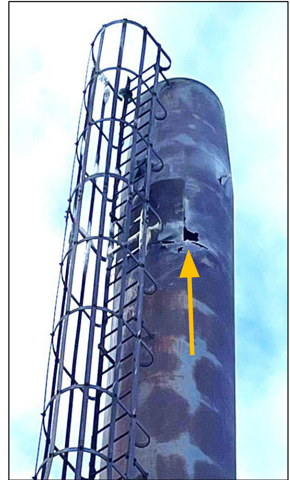
Stack completely rusted through
