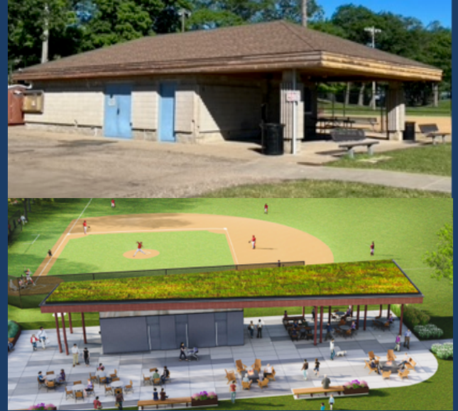
Before & After Photos of the Concession/Plaza (Underway - Estimated to be completed in 2023)
