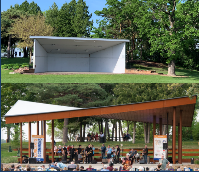
Before & After Photos of the Pavilion (Completed in 2021)
