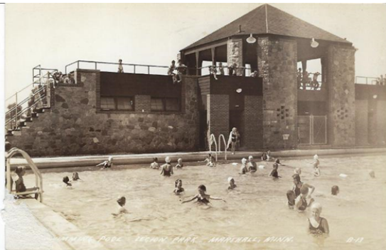
The original 1937-38 constructed Marshall Pool. The Main Pool is still in use today.
