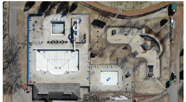
The current 1969 reconstructed facility is showing its age and has numerous deficiencies in code compliance, operations, customer experience and maintenance costs.
