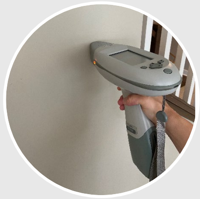
XRF of deteriorated paint
