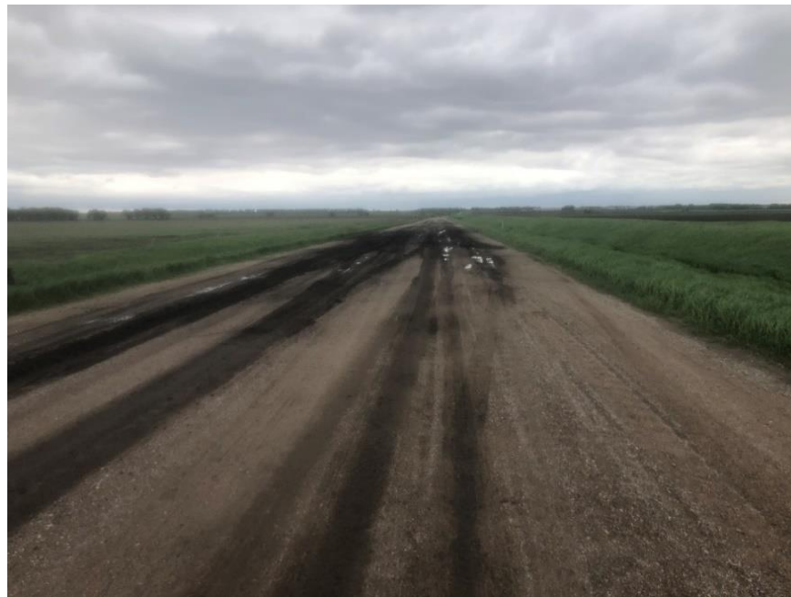
May 31, 2022, 70 th Ave. North condition with no trucks last Spring
