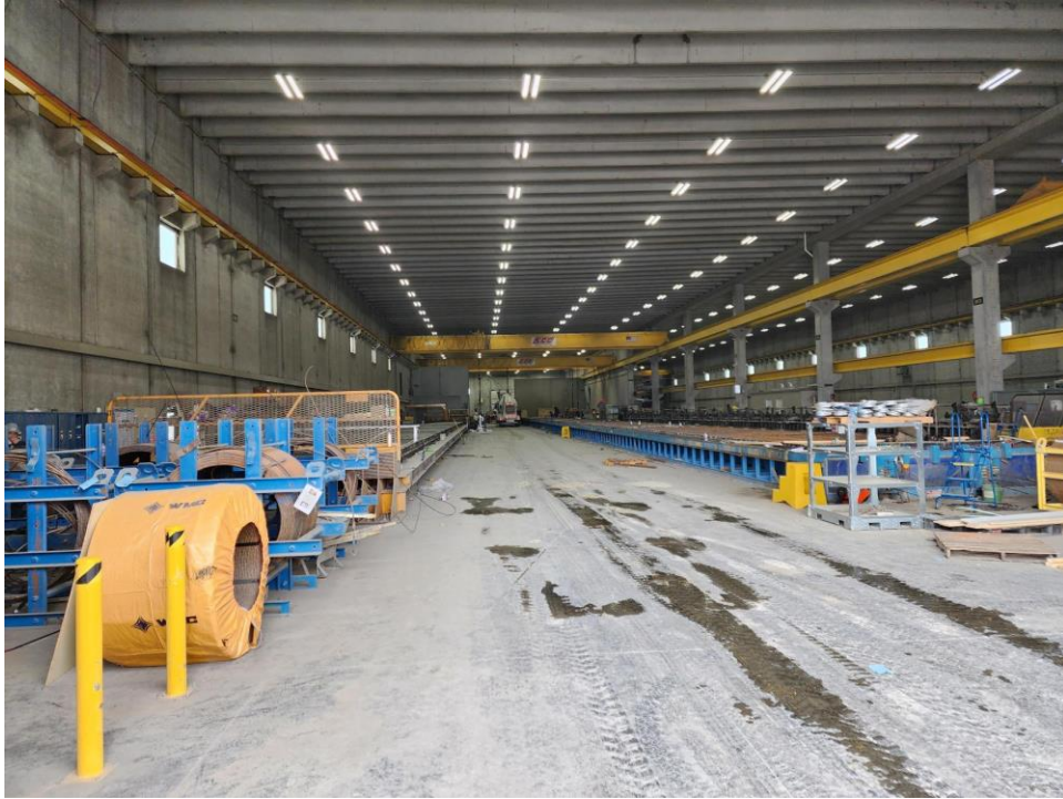
Building 2 Taracon precast production
