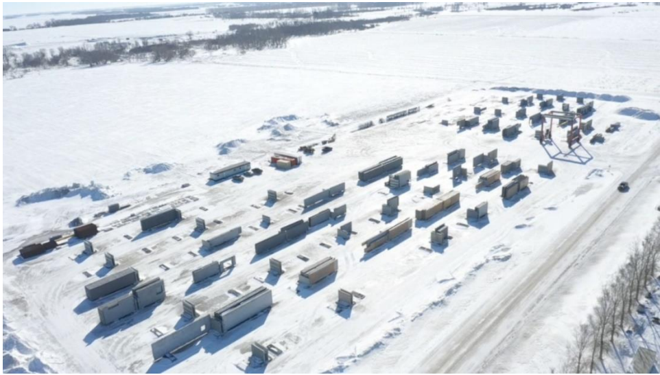
Southeast view of wall staging yard and offices
