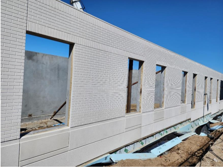
Installation of Polished Precast Concrete Brick Exterior Wall Panels
