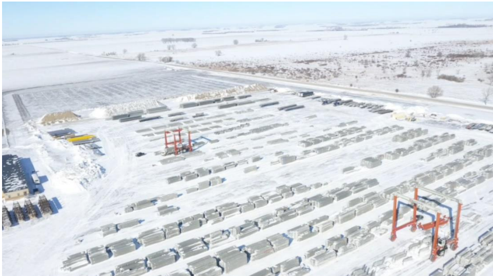
Northwest view of yard at 70th Ave N.
