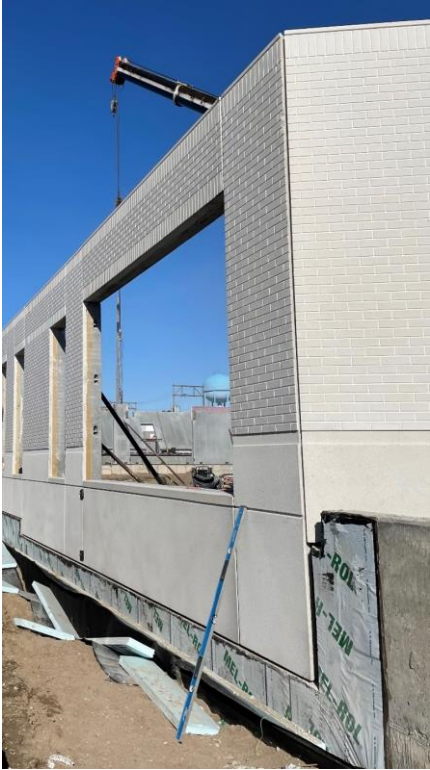
Installation of Polished Precast Concrete Brick Exterior Wall Panels
