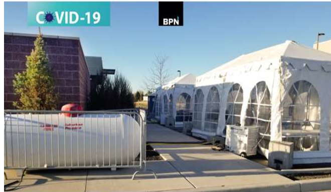
North tent at St. Luke's hospital, Twin Falls, Idaho, fueled by Suburban Propane.
