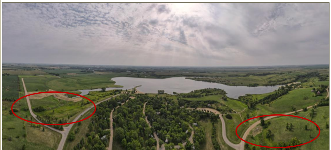
DEL CLARK LAKE GRADE STABILIZATIONS AND ROAD RETENTION (Yellow Medicine County, 2021)
