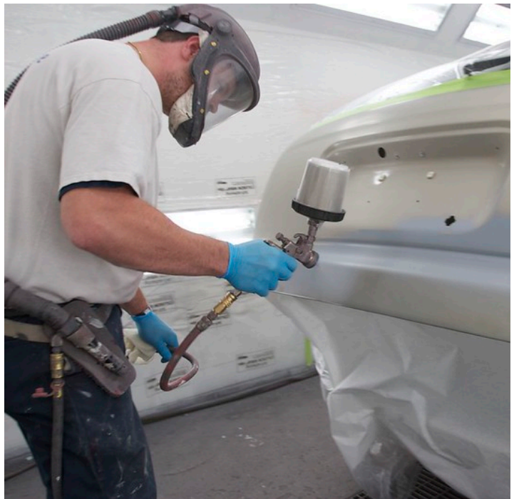
The MPCA has helped auto bodies shops in Minnesota reduce air pollution by adopting water-borne finish systems that work faster with less waste and energy consumption.
