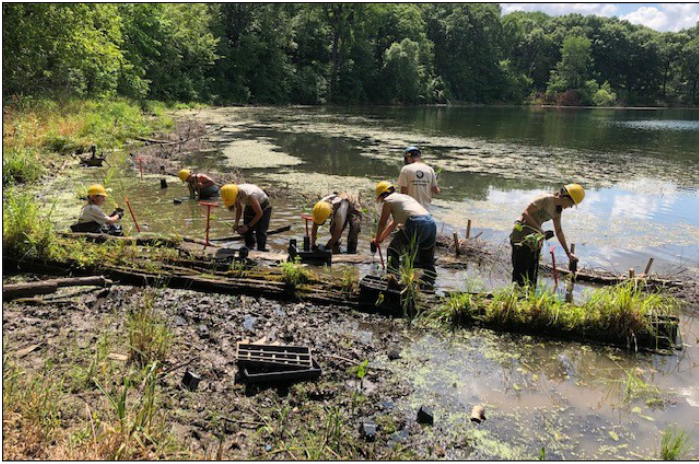
Dakota County Holland Lake Shoreline and Upland Restoration
