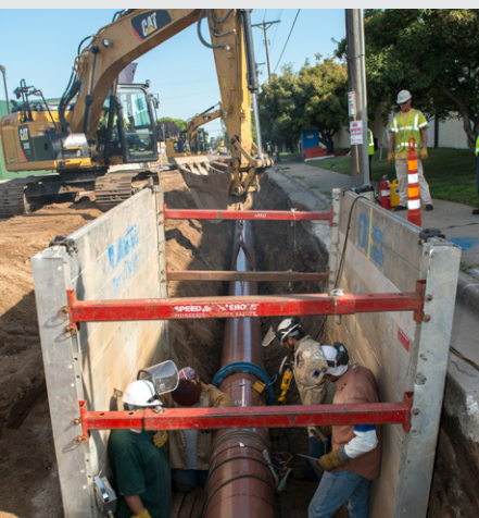
Upgrading our system with durable, state-of-the-art pipeline materials
