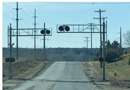
Several unimproved railroad crossings intersect 117th Street, creating additional traffic hazards.
