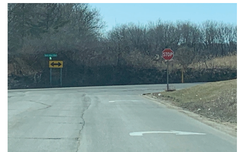
117th currently dead ends into Rich Valley Boulevard, another busy thoroughfare, where trucks must turn into traffic after stopping at a stop sign. The proposed project will realign this intersection and reduce turning movements.
